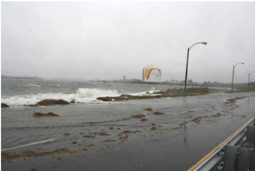
Morrissey Blvd flooding during Hurricane Sandy
