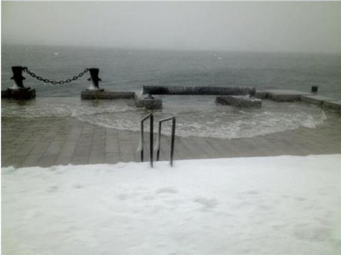
Storm Surge at Long Wharf, February 2013
