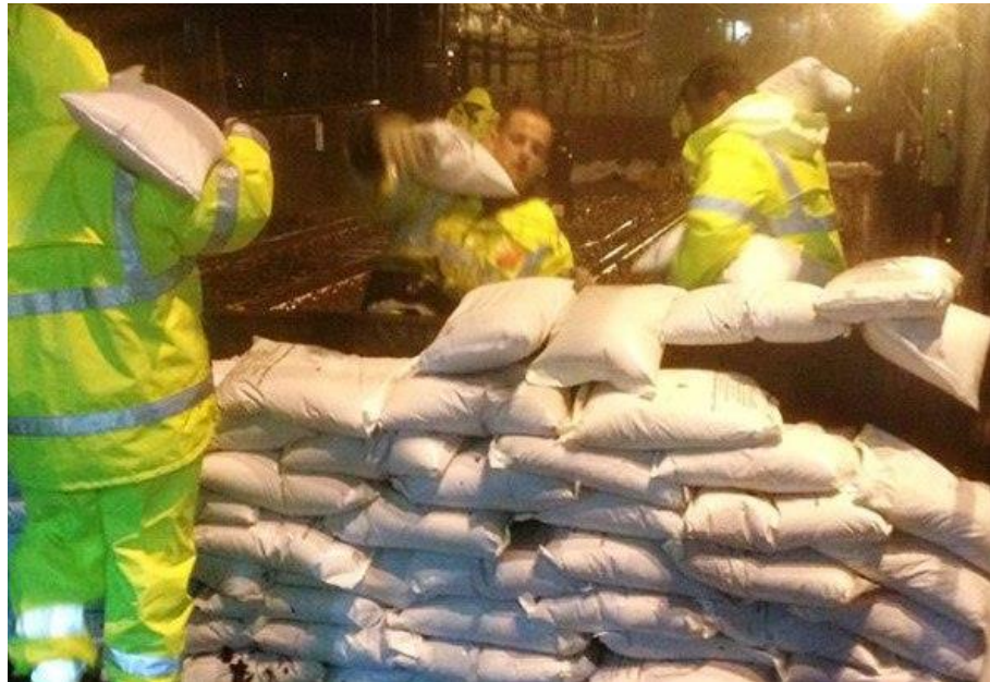
MBTA Workers deploying sandbags at the Green Line tunnel (MBTA photo)
