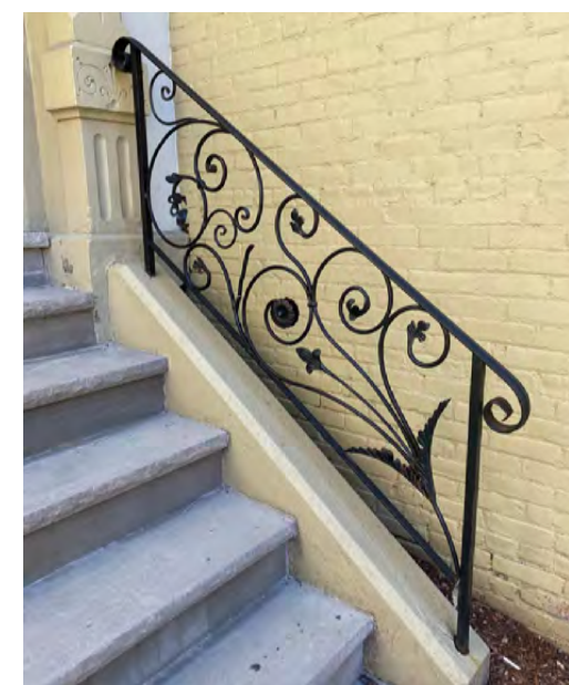
1615 Tremont St – East Railing
