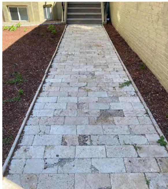
1615 Tremont St – Front Walkway
