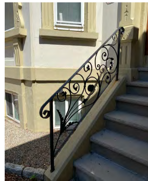
1615 Tremont St – West Railing
