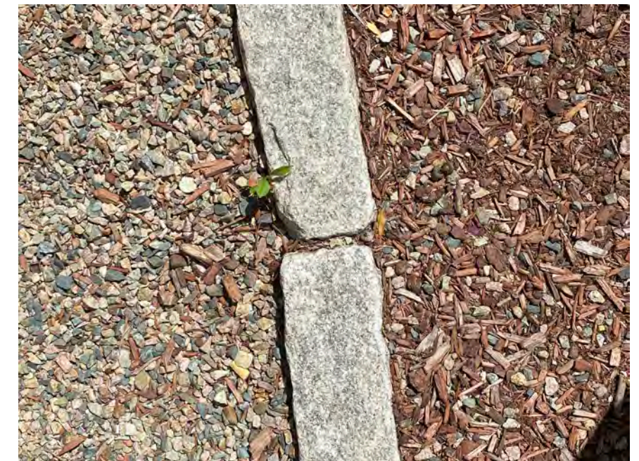
1615 Tremont St – Yard Materials
