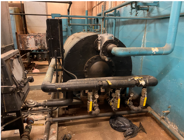
Photos 7: Existing condensate recovery tank and boiler feed unit.
