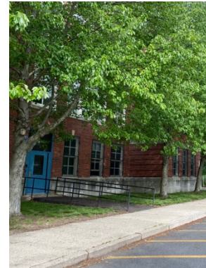
Current Accessible Entry
