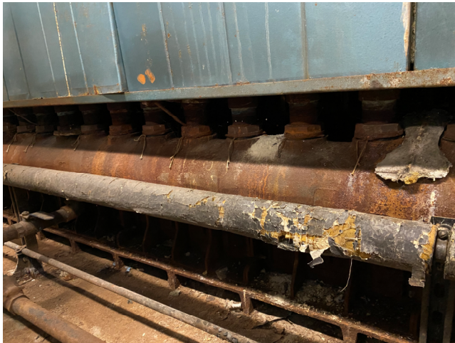
Photos 3 & 4: Existing return headers under the boiler.
