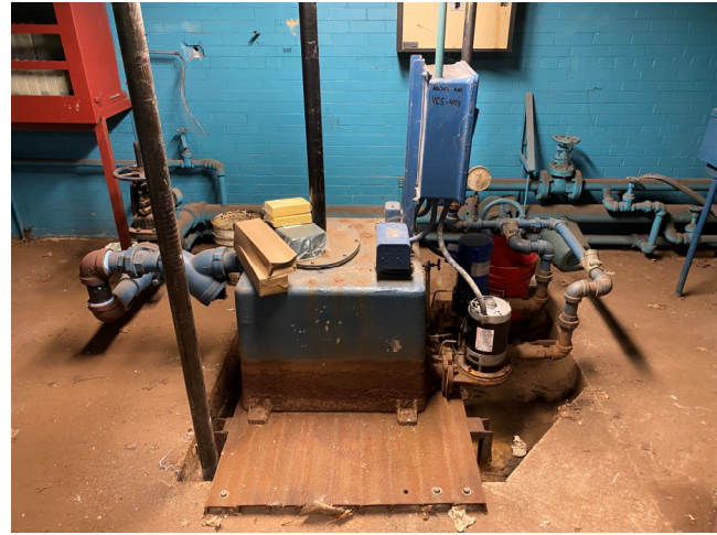
Photos 7: Existing condensate recovery tank and boiler feed unit.
