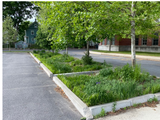
Existing Rain Garden
