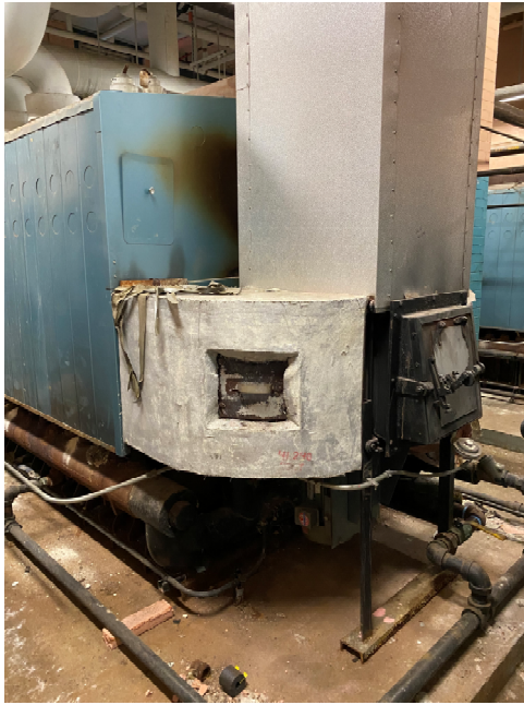
Photos 5 & 6: Existing boiler flue exhaust inducer fan section.
