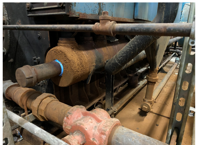
Photos 3 & 4: Existing return headers under the boiler.
