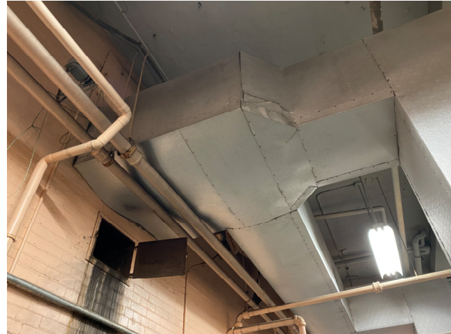
Photos 5 & 6: Existing boiler flue exhaust inducer fan section.
