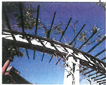
radial metal shade trellis
