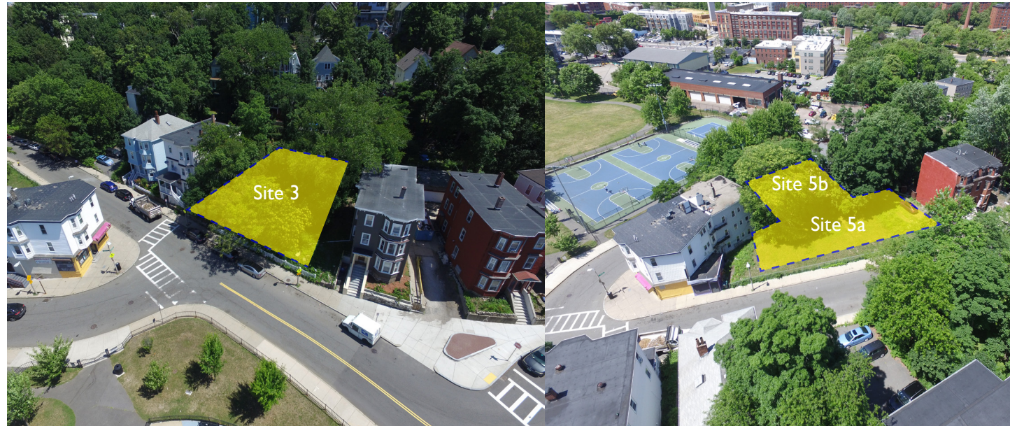
Existing Site Condition
