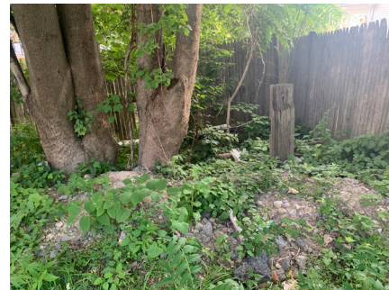
Remnants of former Buildings on-site
