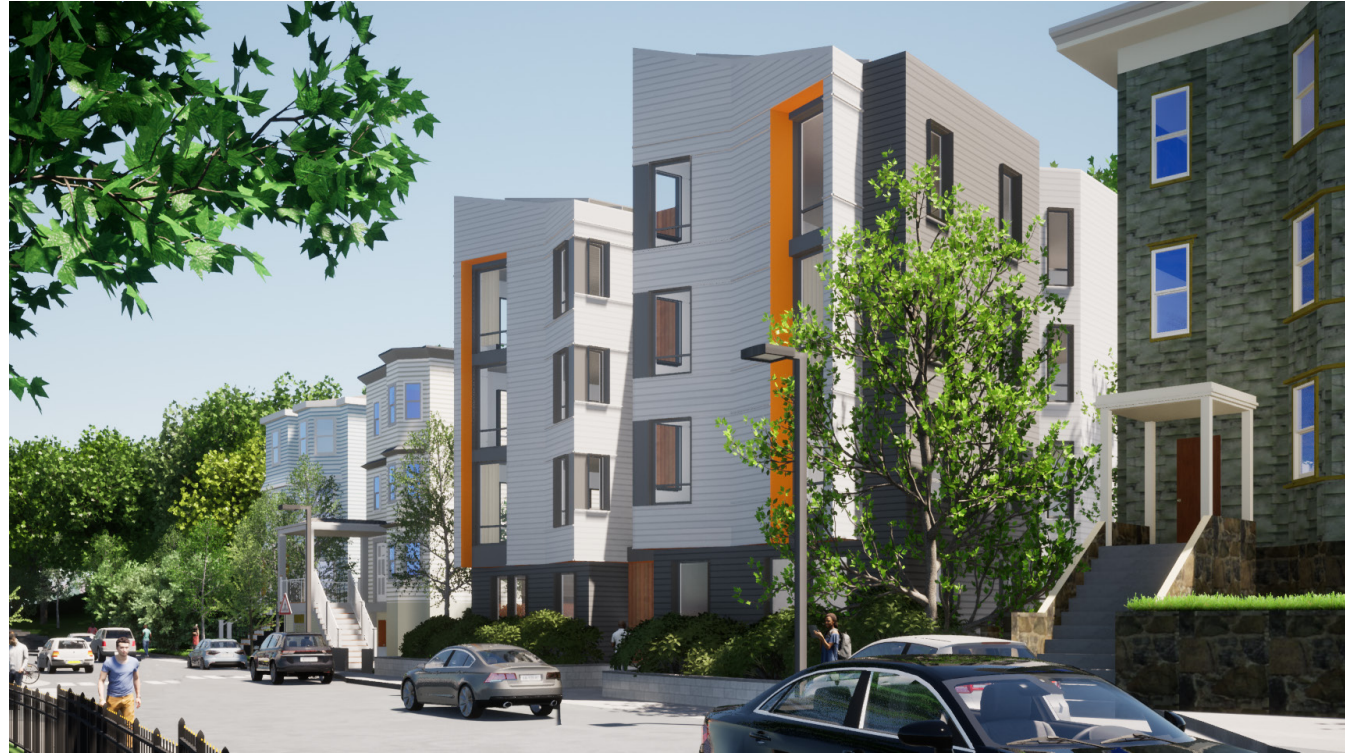
Site 3 - Looking North on Marcella St.
