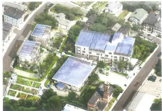
E+ Parker Terrace Solar Arrays / Studio G Architects
