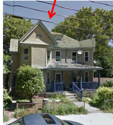
Gable Roof Shape on Bowdoin Terrace
