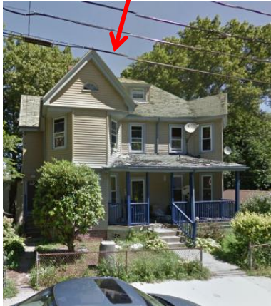
Gable and Hip Roof Shape on Bowdoin Terrace
