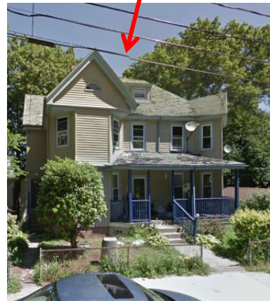
Gable Roof Shape on Bowdoin Terrace
