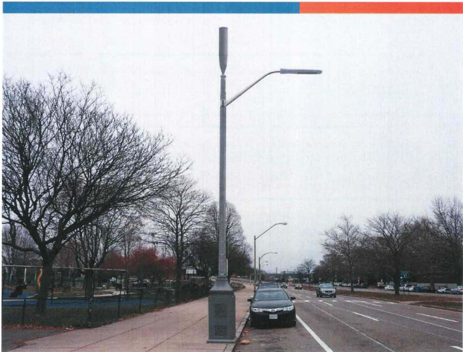
Proposed Conditions: Standard concrete light pole replacement with antenna & equipment enclosure.
