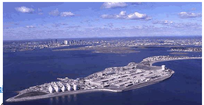
Deer Island Waste Water Treatment Plant
