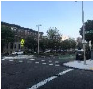
**Constructed curb extensions and extended the median to create pedestrian refuge space** for the crossing of Brighton Avenue at Chester Street.
