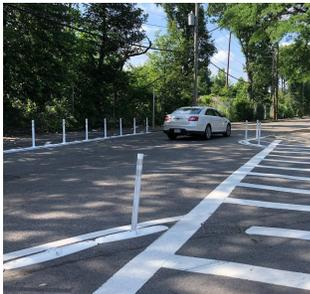
**Installed temporary curb extensions** using pavement markings and flex posts at New England Avenue and Southern Avenue in the Talbot Norfolk Triangle.
