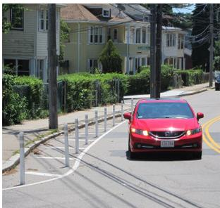
**Used pavement markings and flex posts to better guide vehicles through a curve** approaching the intersection on Wood Avenue near Mariposa Street in Mattapan.
