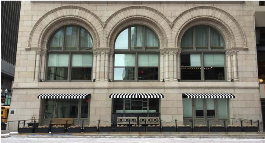
PROPOSED AWNING | OPTION 1: SUNBRELLA FABRIC COLOR TO BE BLACK AND WHITE VERTICAL STRIPES. THE NAME OF THE RESTAURANT WILL NOT BE ON FRONT OF AWNINGS.
