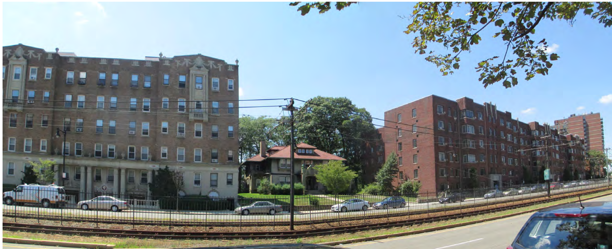
EXISTING CONDITIONS PHOTOS
