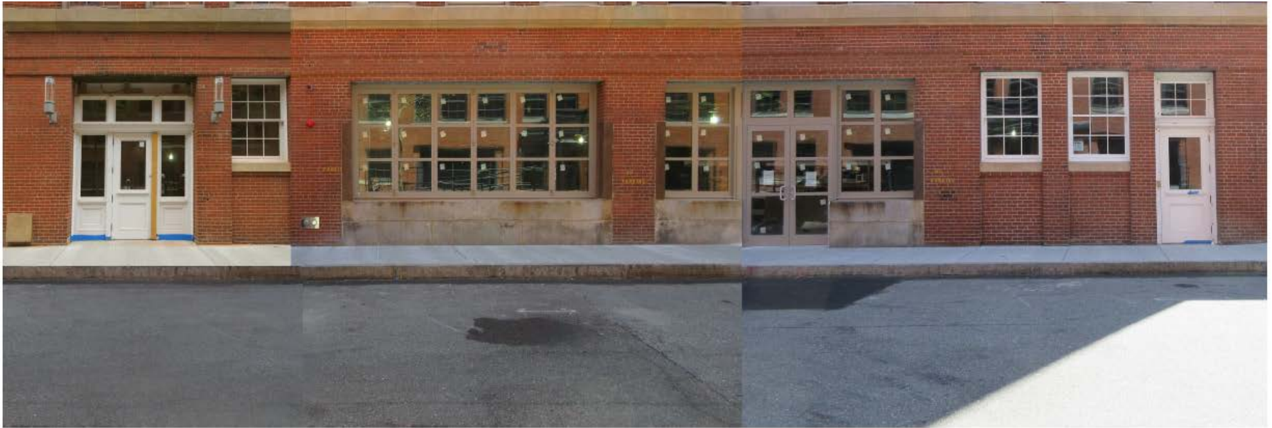
1 COMBINED PROGRESS PHOTOGRAPHS OF WEST FACADE
