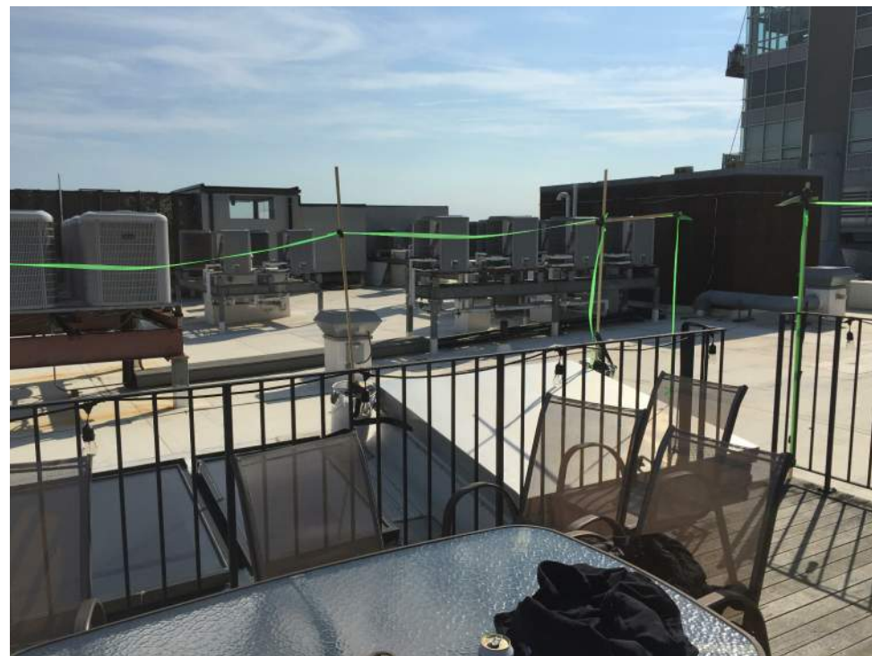
02 - SOUTH-EAST VIEW OF HATCH ENTRY - MOCK-UP RAILING AND WALL INSTALLED
