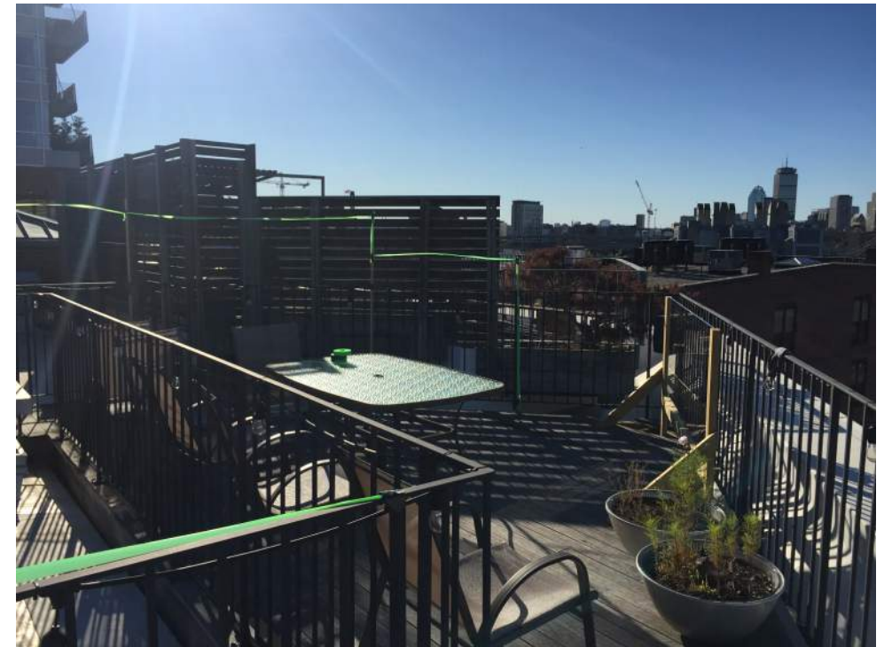
04 - SOUTH VIEW OF LOUNGE AREA - MOCK-UP RAILING AND WALL INSTALLED
