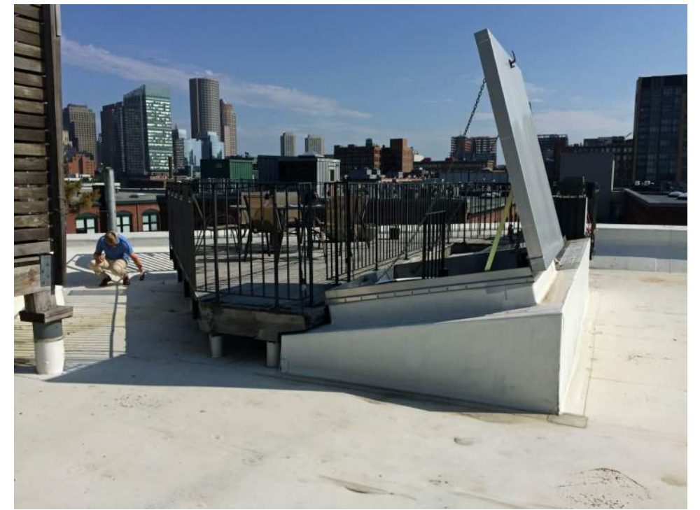
03 - NORTH VIEW OF HATCH OPENING
