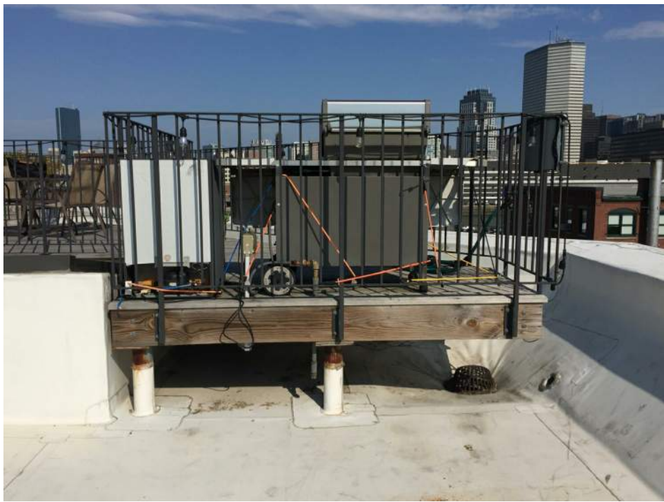
01 - NORTH-WEST VIEW OF EXISTING GRILL AREA
