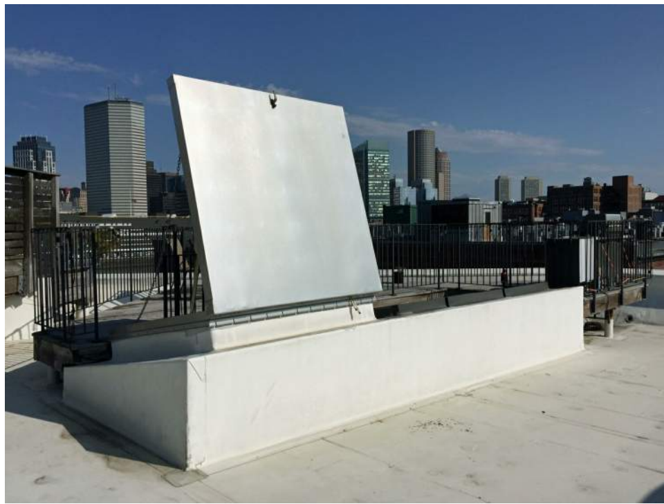
02 - NORTH VIEW OF EXISTING HEAD HOUSE
