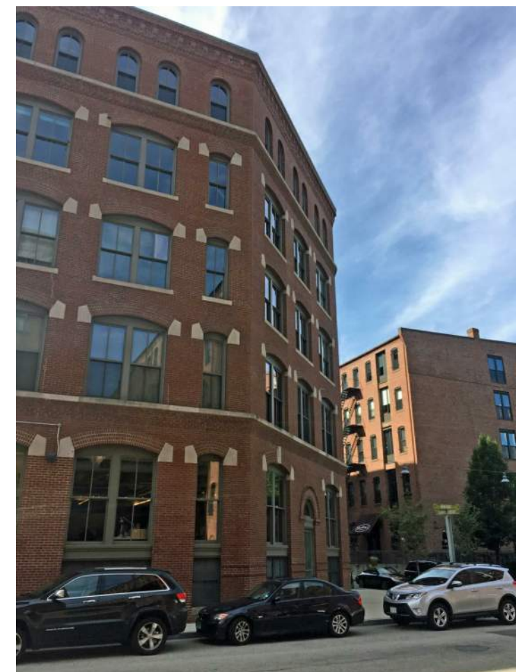
06 - SOUTH VIEW FROM BINFORD STREET - AREA OF WORK NOT VISIBLE
