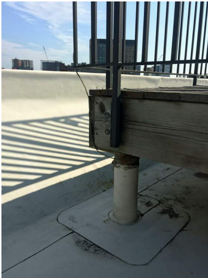
04 - VIEW OF EXISTING DECK STRUCTURE
