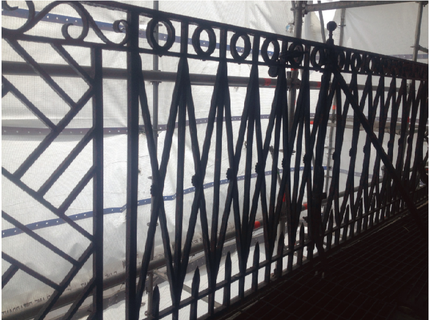
PARTIAL SOUTH RAILING
