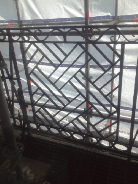
PARTIAL SOUTH RAILING
