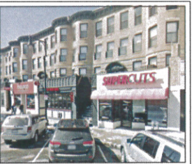
N/W BEACON STREET STARBUCKS AND PIZZA ON OTHER SIDE OF RENOVATION SPACE METAL STOREFRONTS ON STONE VENEER ON WOOD BASE PAINTED EXPOSED HISTORIC PARAPETS
