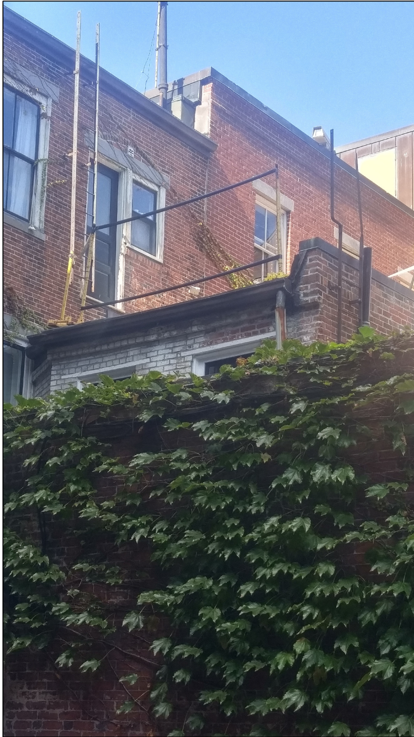
9. Photo of mock-up from Ridgeway Lane
