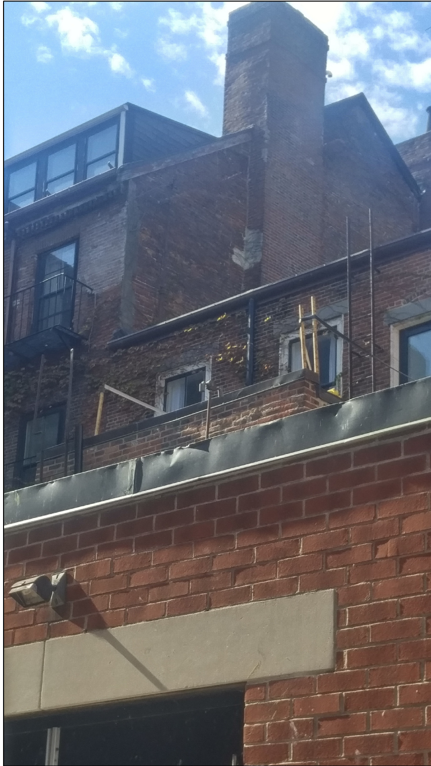
10. Photo of mock-up from Ridgeway Lane
