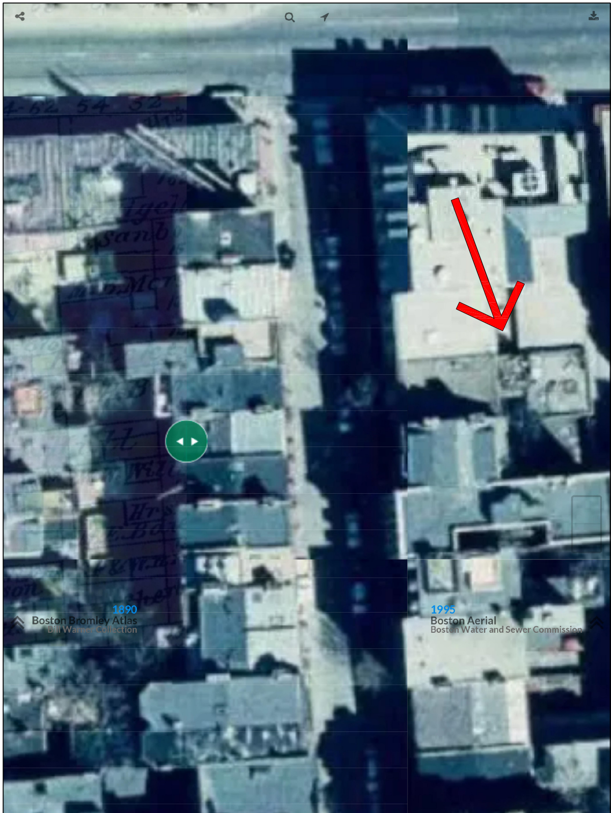
1. Aerial photo showing pre-existing roof deck
