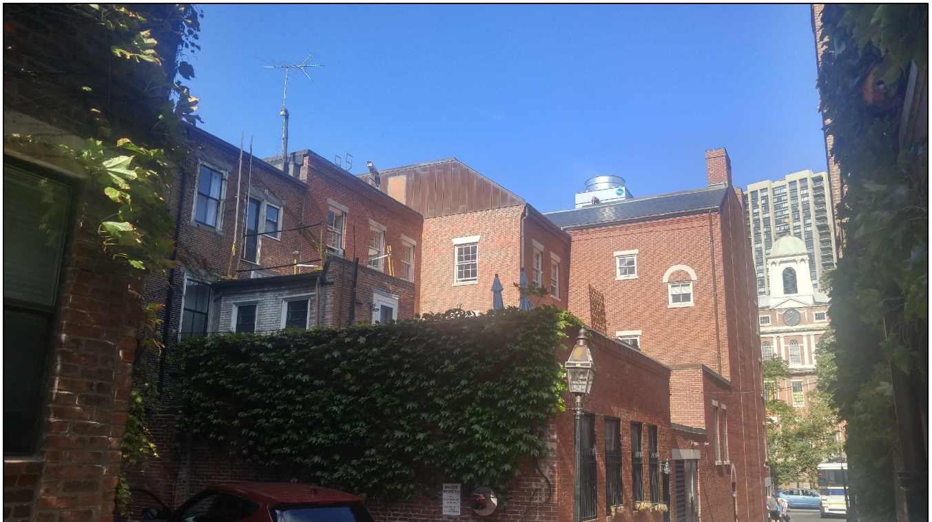
8. Photo of mock-up from Ridgeway Lane
