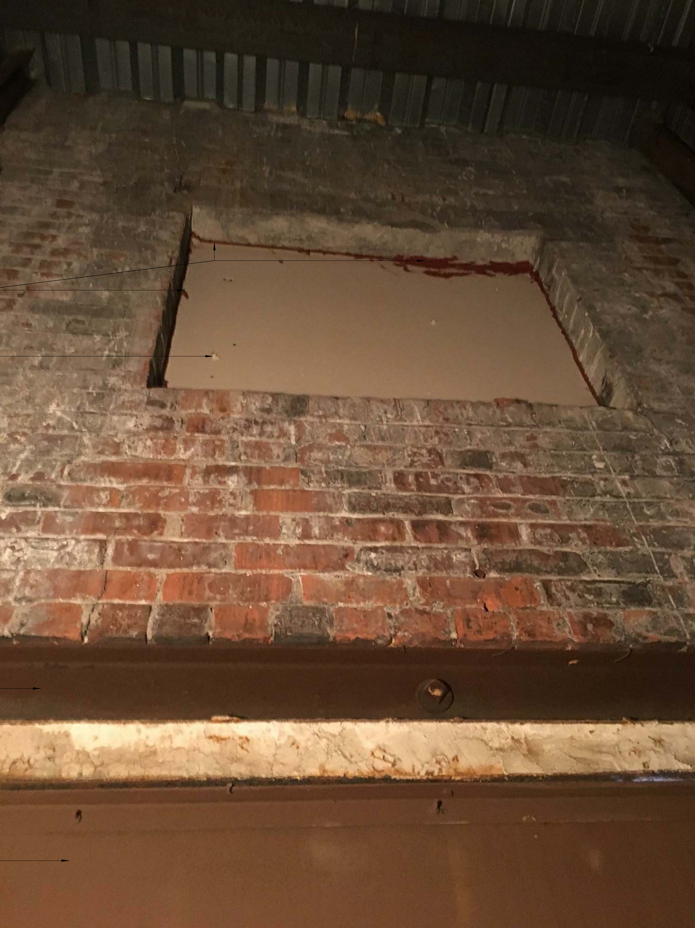
INTERIOR PHOTO @ PANELED OFF MASONRY OPENING
