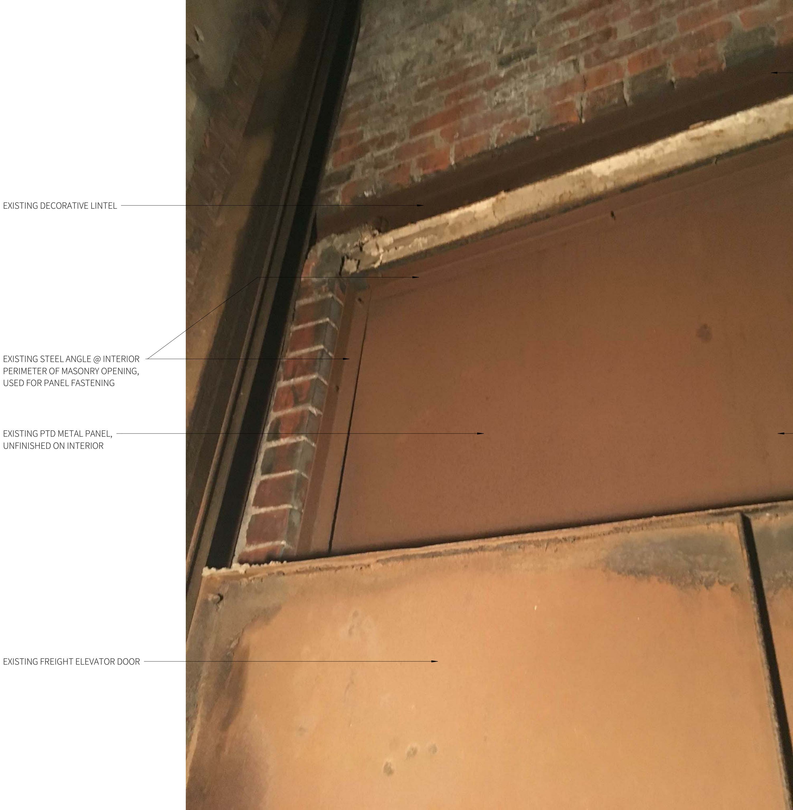
INTERIOR PHOTO @ MTL PANEL ABOVE FREIGHT ELEVATOR DOOR
