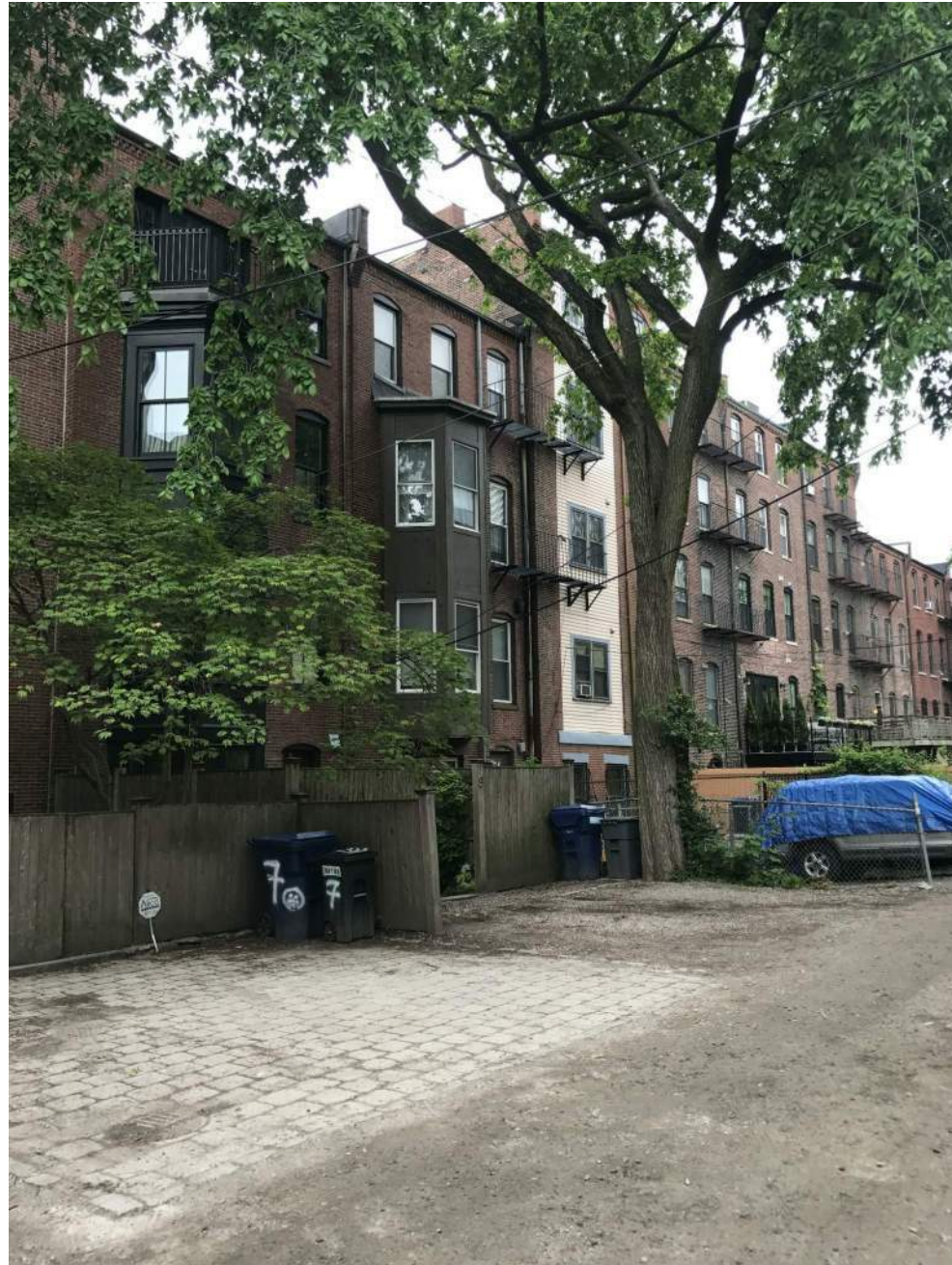
REAR ALLEY FACING NORTH
