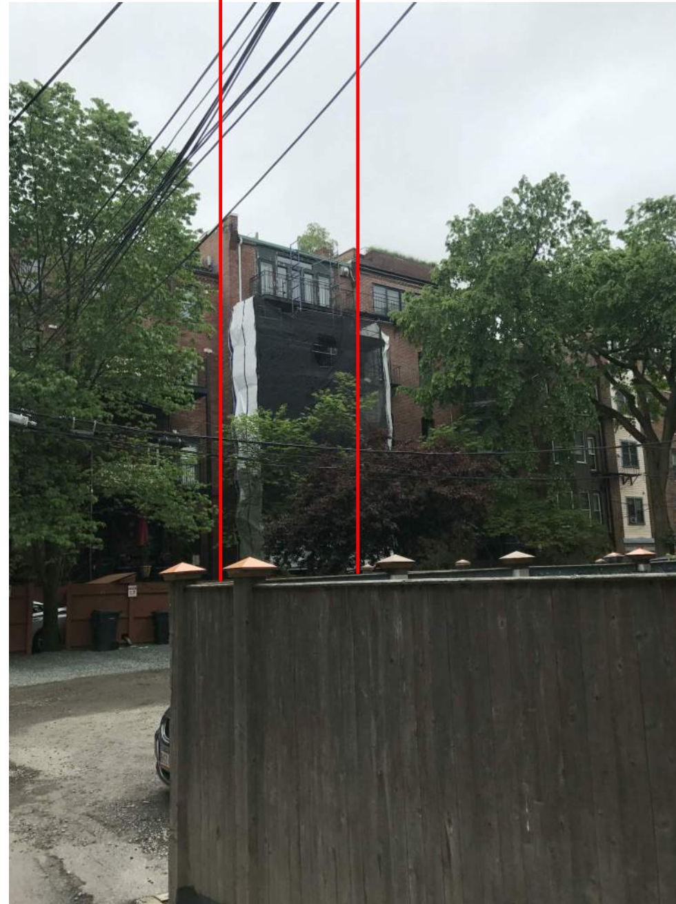
CURRENT CONDITION OF REAR ELEVATION - 5 CLAREMONT PARK
