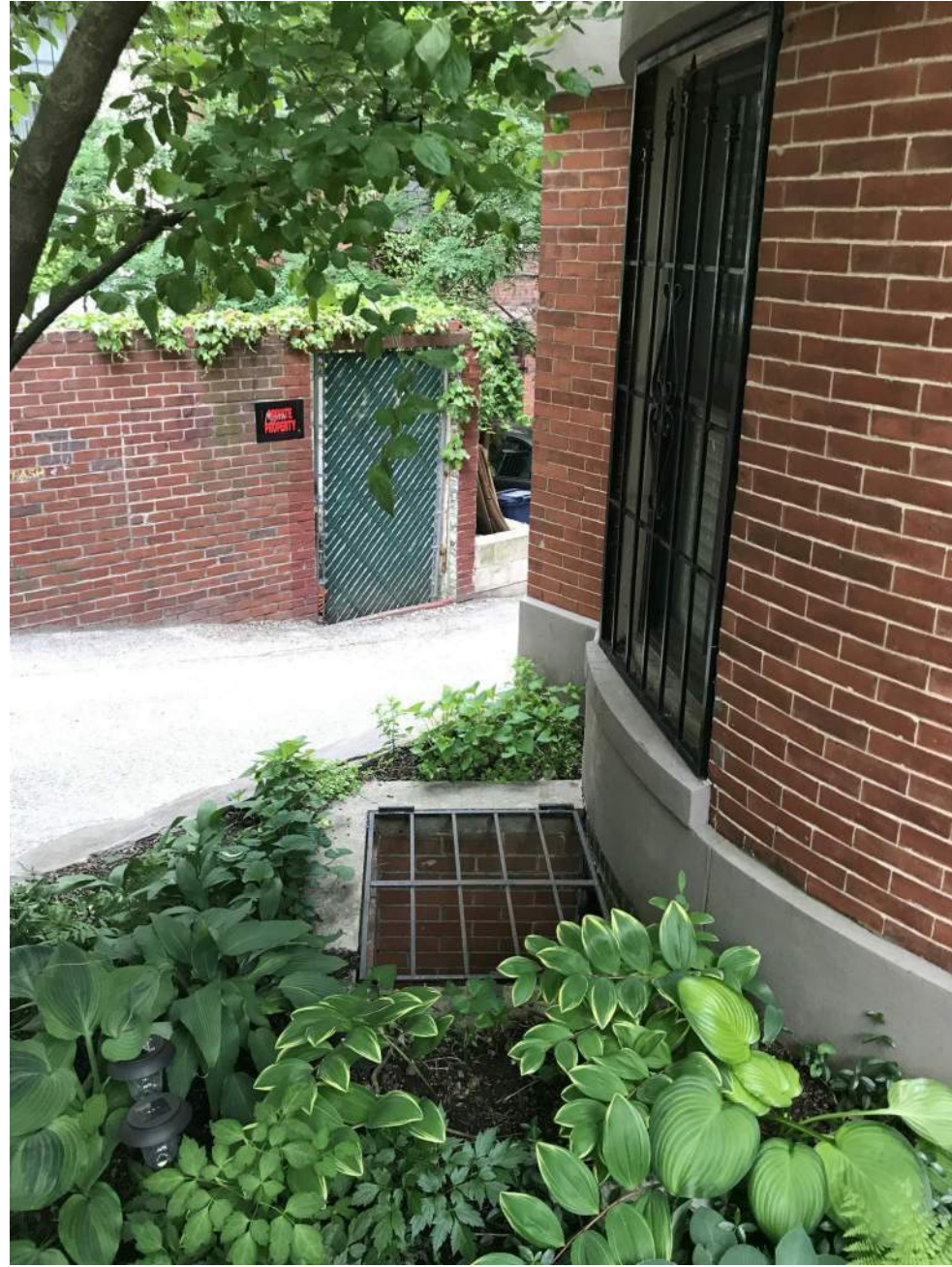
WINDOW WELL AT 2 CLAREMONT PARK
