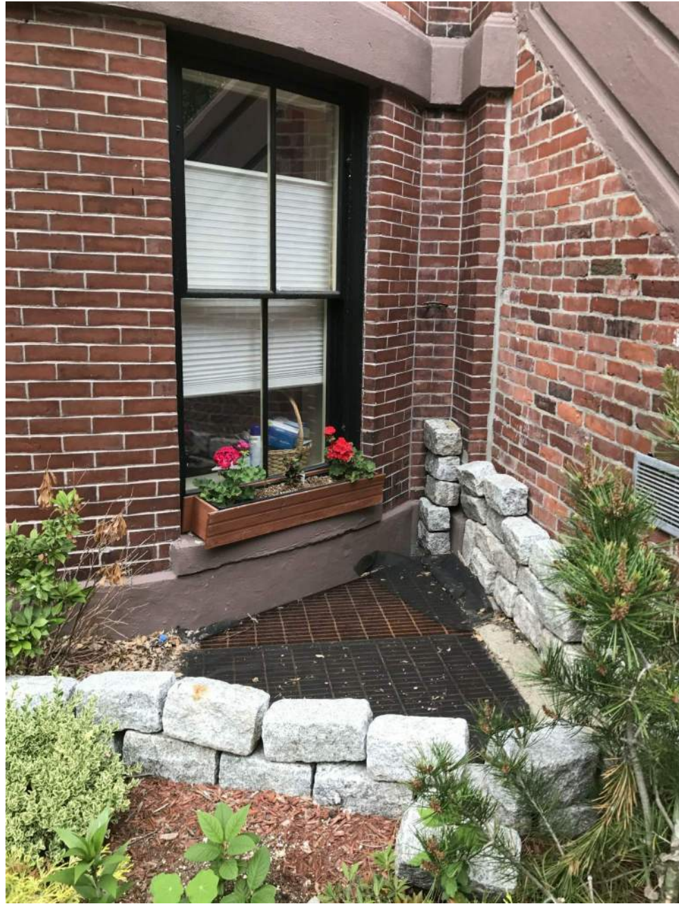
WINDOW WELL AT 3 CLAREMONT PARK
