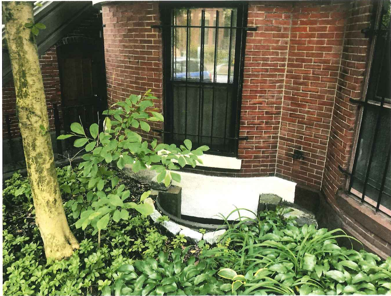
WINDOW WELL AT 12 CLAREMONT PARK
