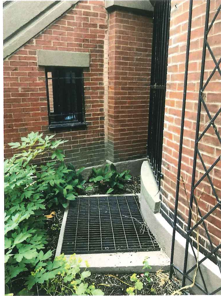
WINDOW WELL AT 4 CLAREMONT PARK
