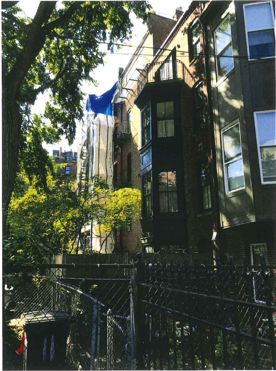
REAR ALLEY FACING SOUTH
