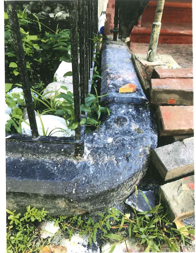
REPAIR EXISTING MASONRY CURB.
