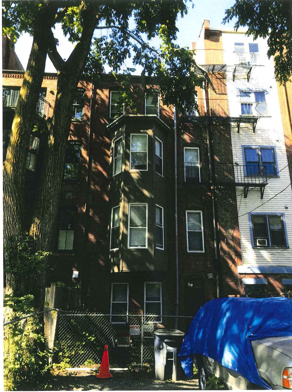
REAR ELEVATION OF 11 CLAREMONT PARK (PRIVATE ALLEY)
