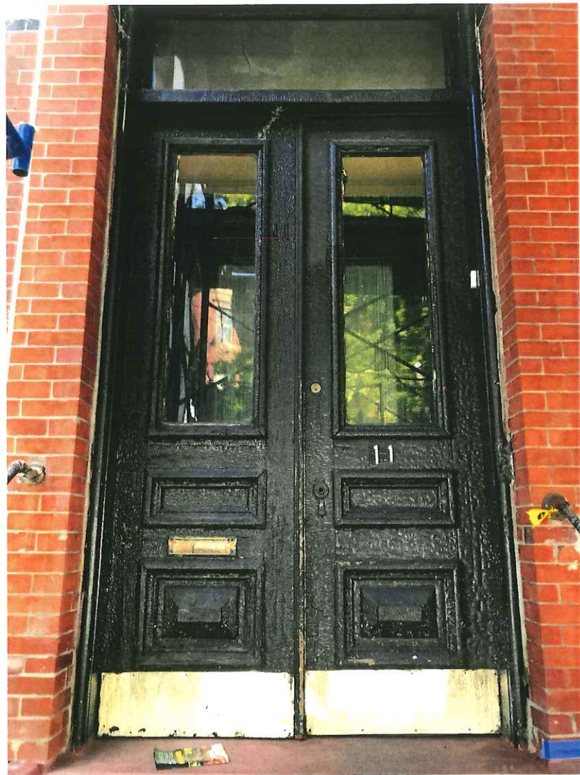
REPAIR AND RESTORE EXISTING FRONT DOOR. INSTALL NEW HARDWARE
