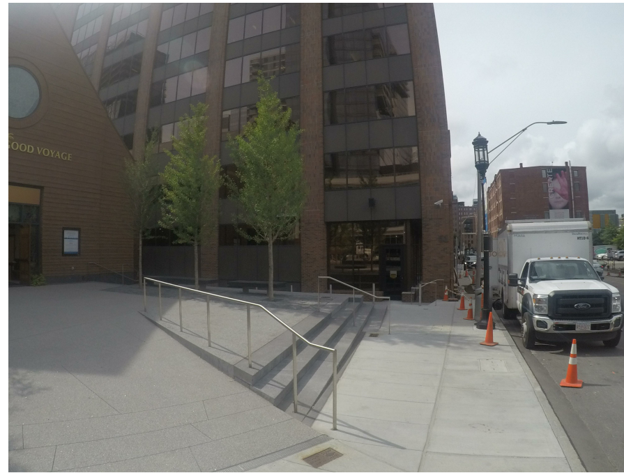
② EXISTING CONDITIONS - CORNER VIEW
