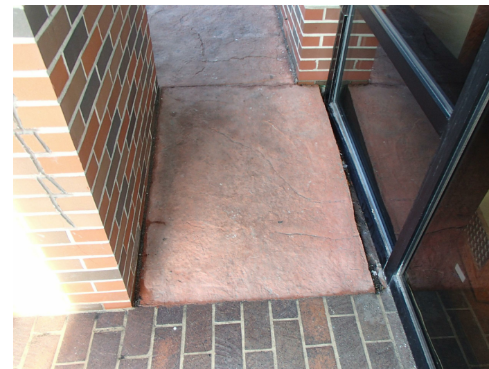
⑥ EXISTING CONDITIONS - PATIO
