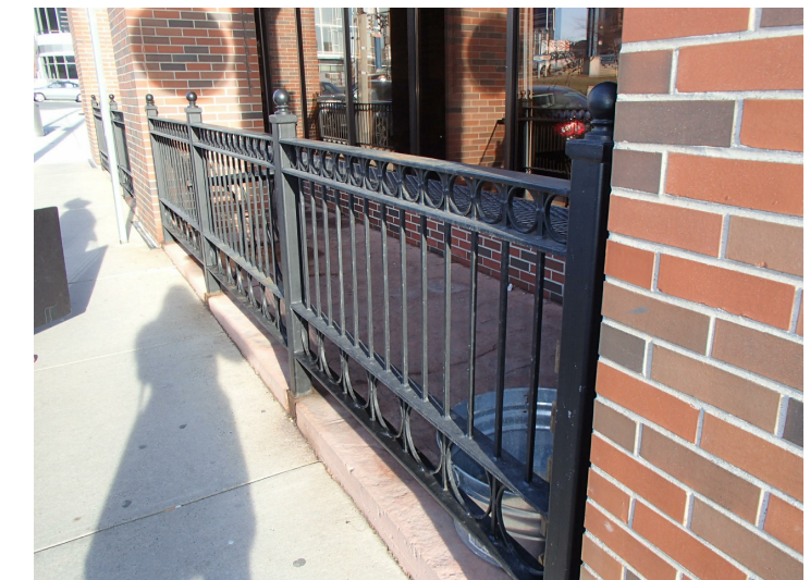
⑦ EXISTING CONDITIONS - PATIO
