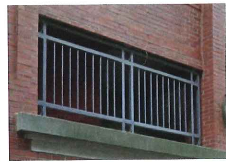
Farnsworth Street Garage
