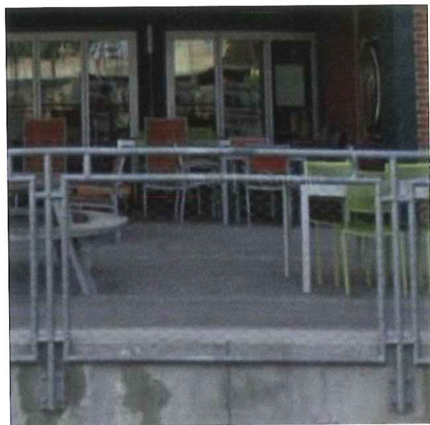
333 Summer Street facing West Service Road
