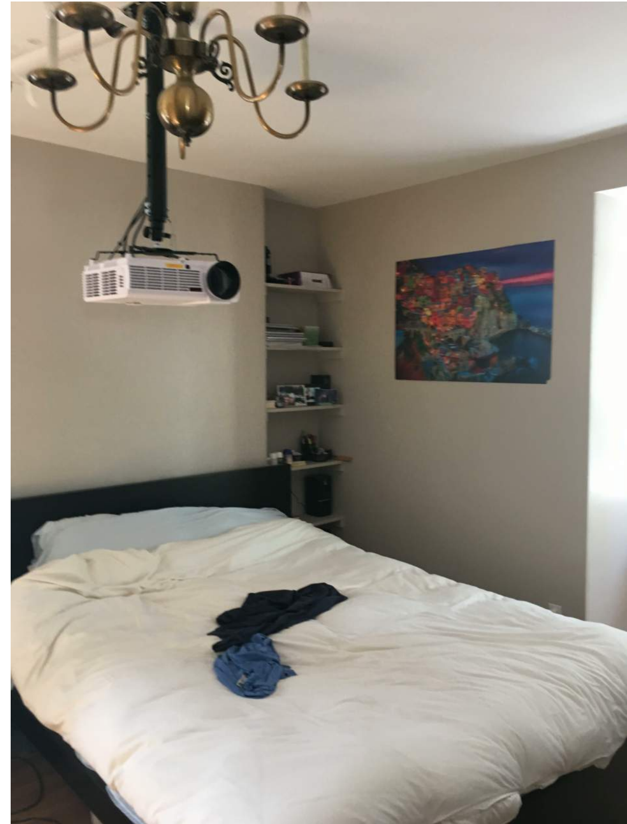
EXISTING CHIMNEY BREAST AT INTERIOR - THIRD FLOOR
