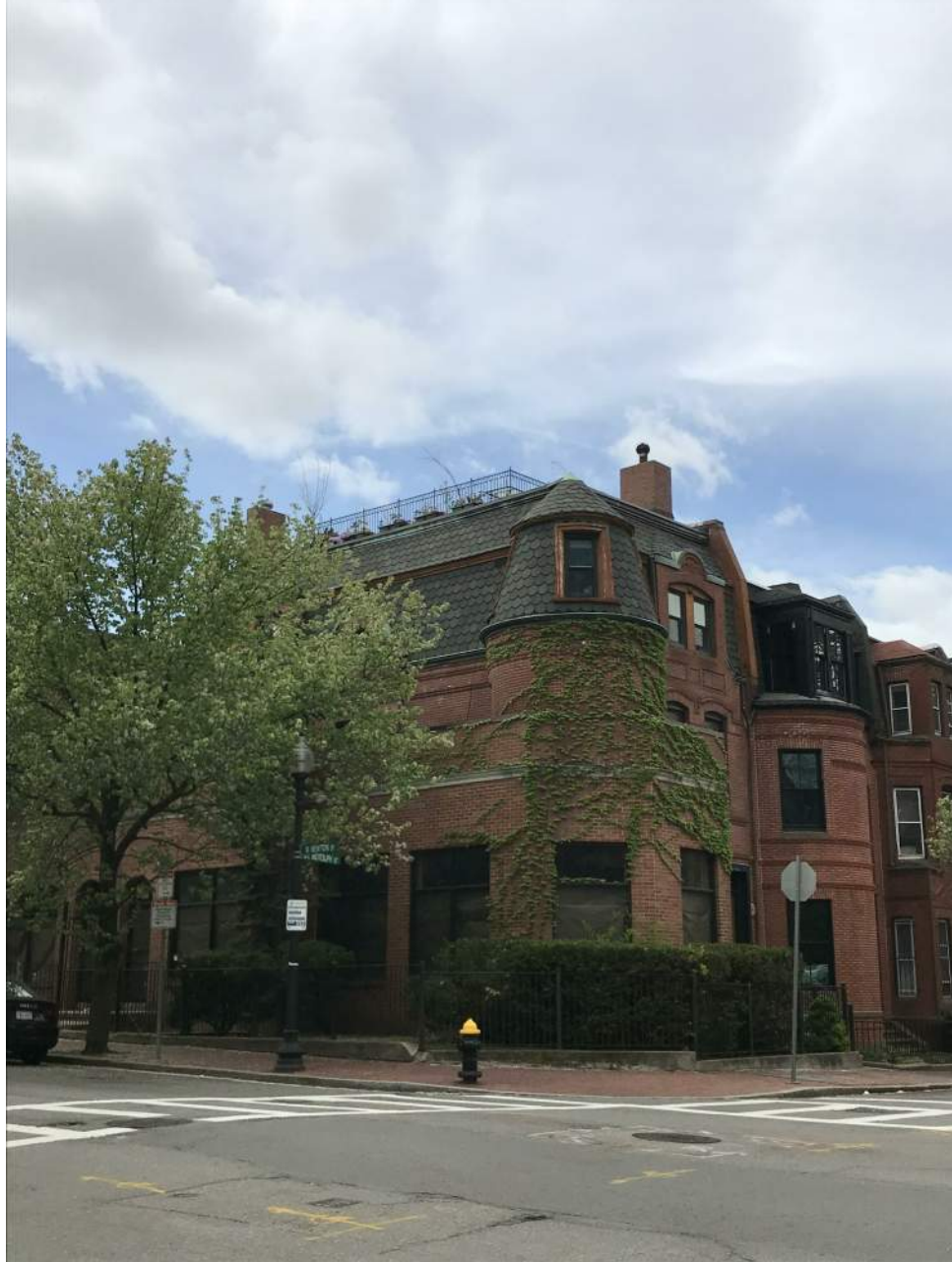
VISIBLE RAILING AT 250 W. NEWTON STREET
