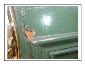
Sample 3: This sample was taken from a crack between molding sections at the top of the lower east panel. It was found to contain only primer and paint.
