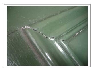
Sample 4: This sample was taken from the middle of the right side of the lower west panel between the panel and the molding. The sample was found to contain only sealant and paint.
