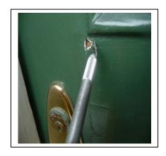
Sample 2: This sample was taken from a "lump" near the lock on the lower part of the sample rail, directly below sample 1. This sample contained only paint. The wood was also friable over a very small area.
