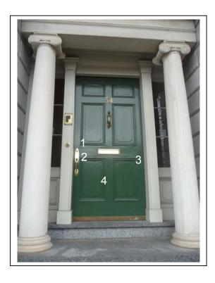
Sample 1: At the left end of the lock rail, top. This sample was found to have a small amount of what appeared to be an epoxy filler, followed by a white primer and the green paint top coat. The wood under the filler was somewhat friable over a small area, less than one square inch
