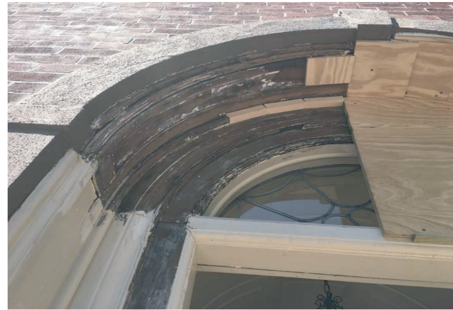
Detail shot of exterior trim for repairs & paint to match existing.
