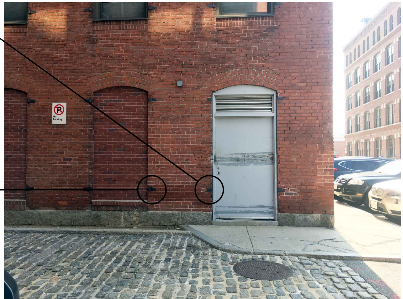
EXISTING TRASH / RECYCLING ROOM DOOR
