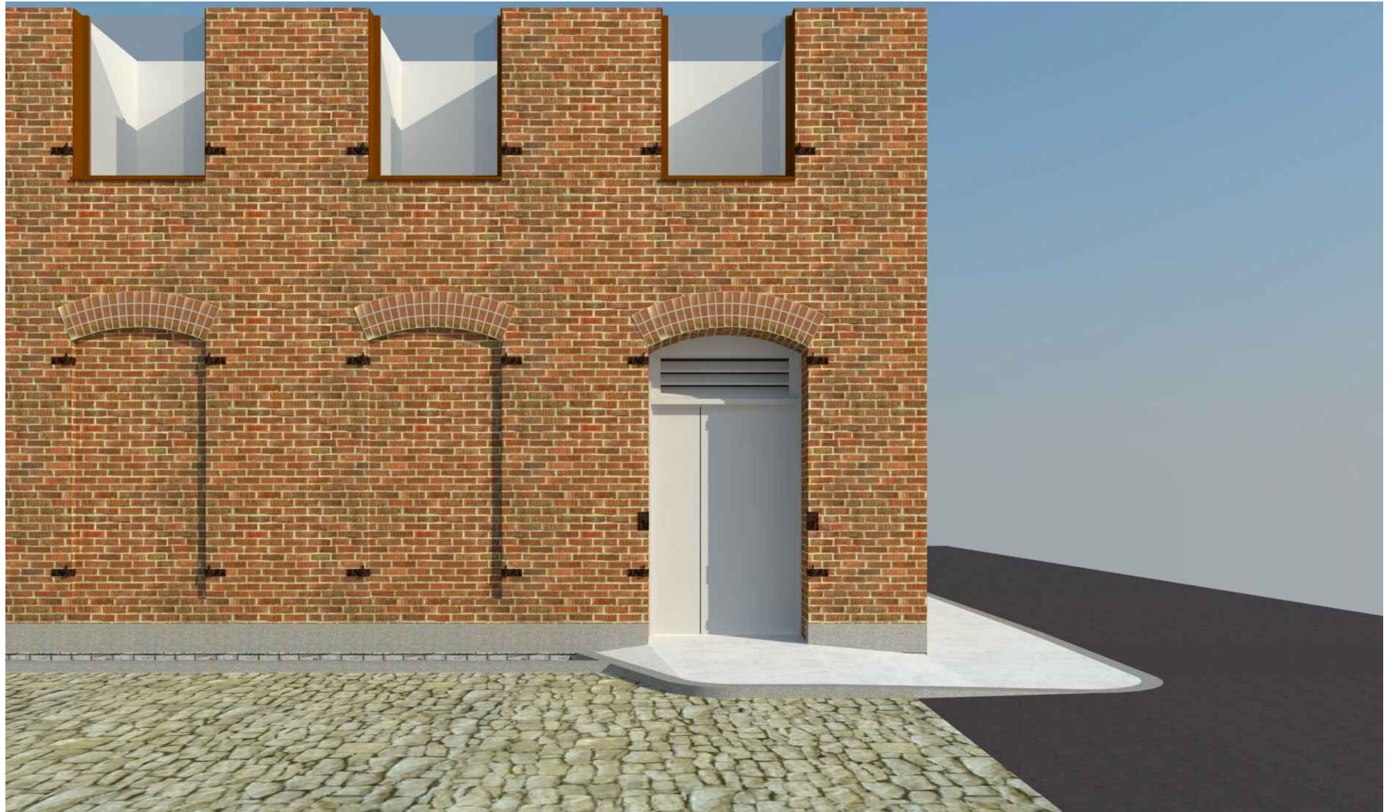
VIEW FROM ACROSS THE ALLEY
