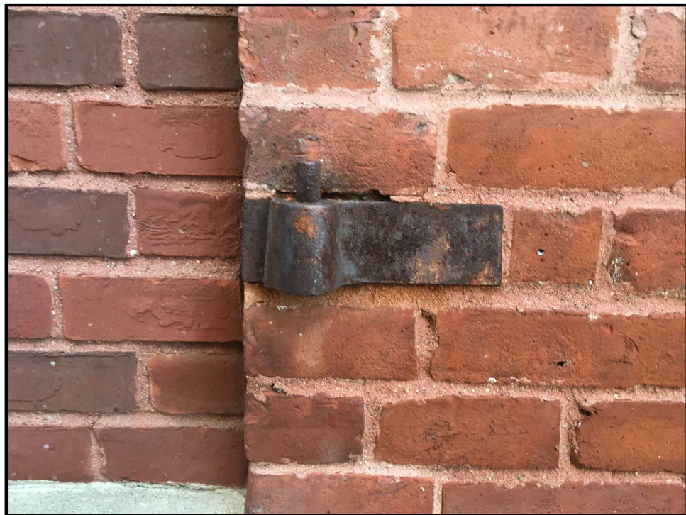
EMBEDDED FIRE SHUTTER HINGE INTACT (TYPICAL)
