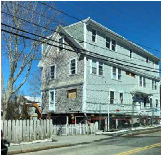
Some homes in the South Boston residential neighborhood along Day Boulevard may be appropriate for elevation in the long term, such as this example of an elevation in progress from Provincetown, Massachusetts.
