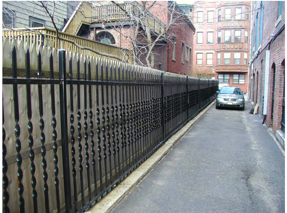
Representative Photo of Iron Fence from Beacon House Side
