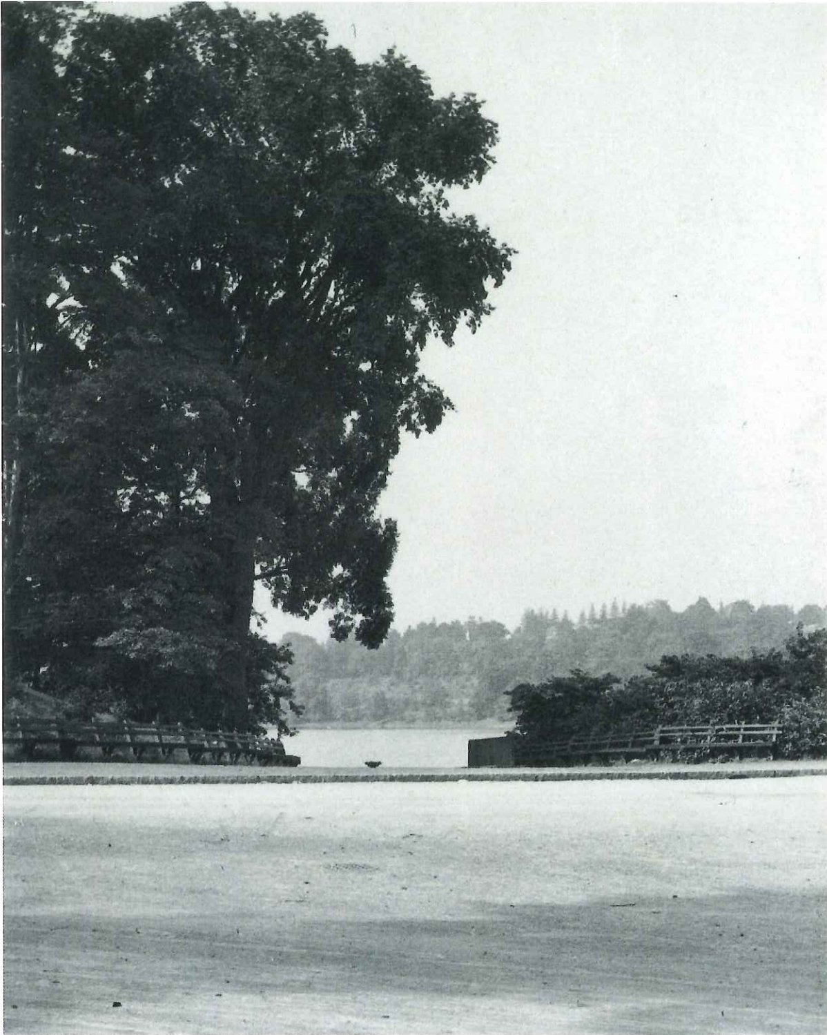
Perkins/Chestnut Street Entry, no date; Courtesy of Olmsted NHS Archives
