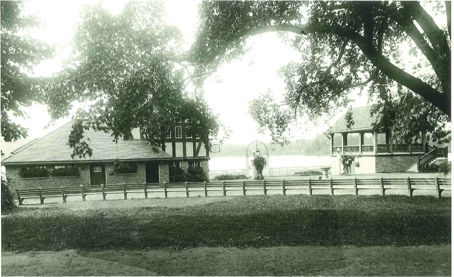
Boathouse & Bandstand, no date; Courtesy of Olmsted NHS Archives
