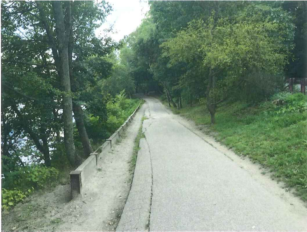
Example of timber retaining wall along perimeter pathway below Perkins Street, 2018
