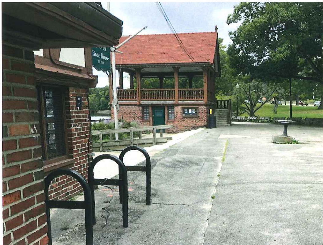
Surrounding landscape at Boathouse/Bandstand plaza. Note: overhead wires, bike racks, and drinking fountain, 2018
