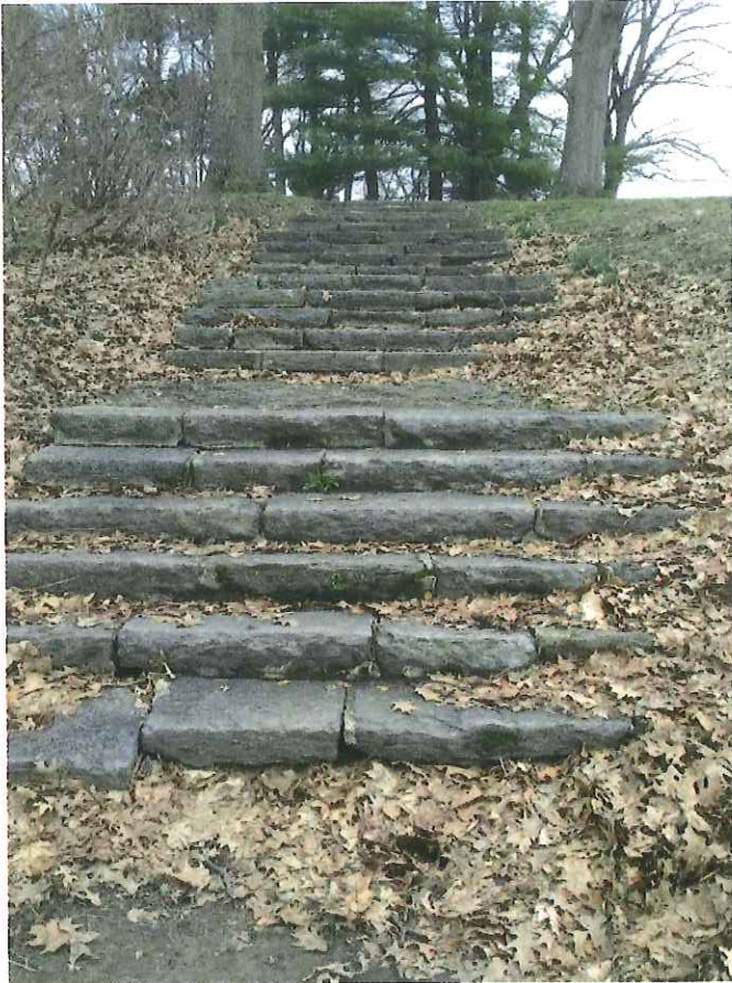
Existing conditions (May)
