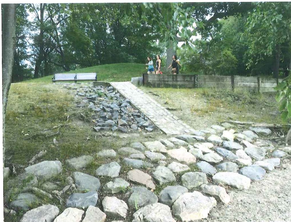
Example of cobblestone spillway below Perkins Street, 2018
