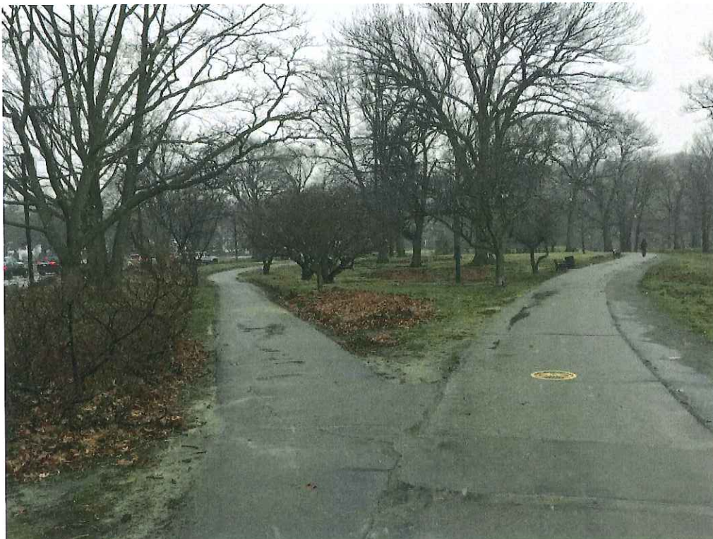
Existing conditions of pathway near the William F. Kelley Circle, 2018
