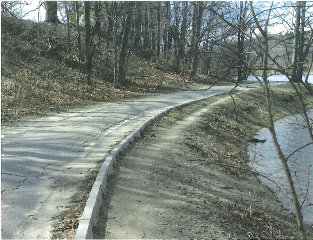
Example of running path inside of vertical granite curb along perimeter pathway below Pinebank, 2018
