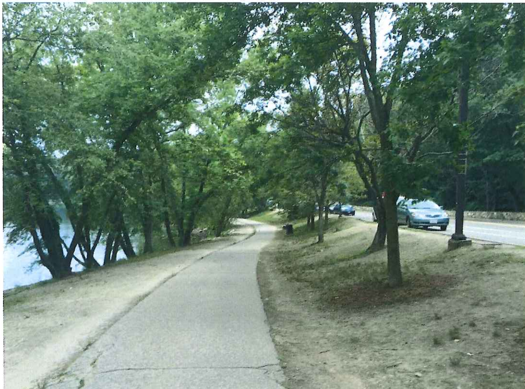
Existing conditions of pathway and slope along Perkins Street, 2018
