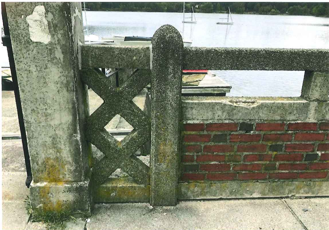
Concrete & brick “fence” at Boathouse/Bandstand plaza, 2018
