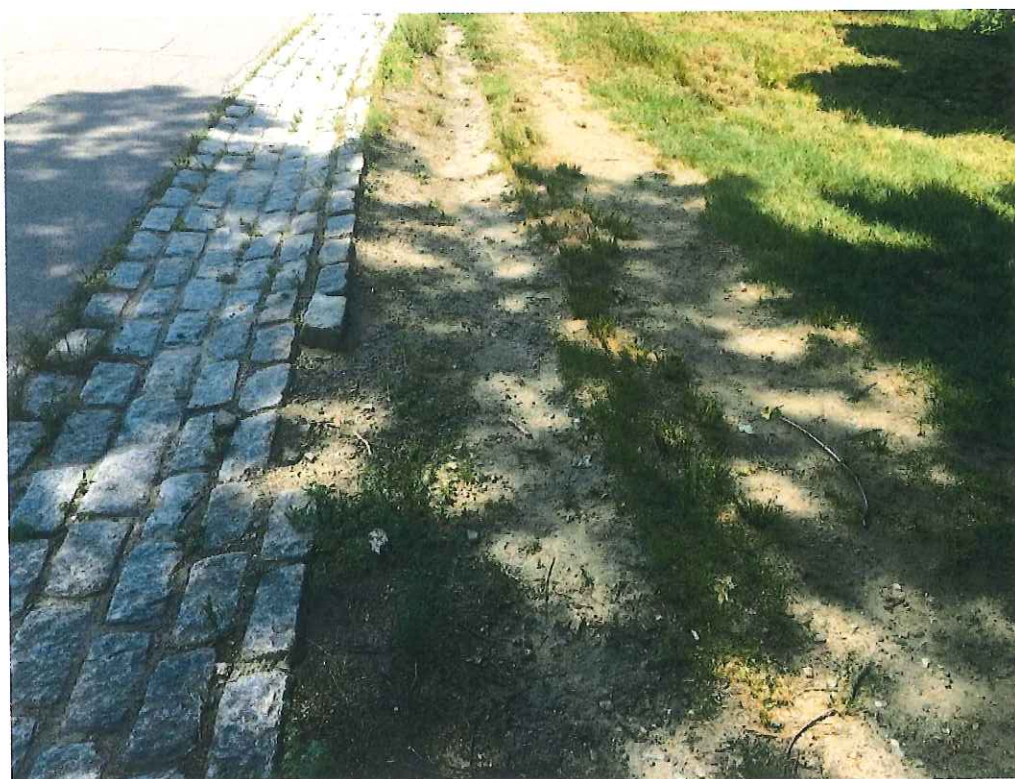
Example of cobblestone swale running parallel to perimeter path along the Jamaicaway, 2018
