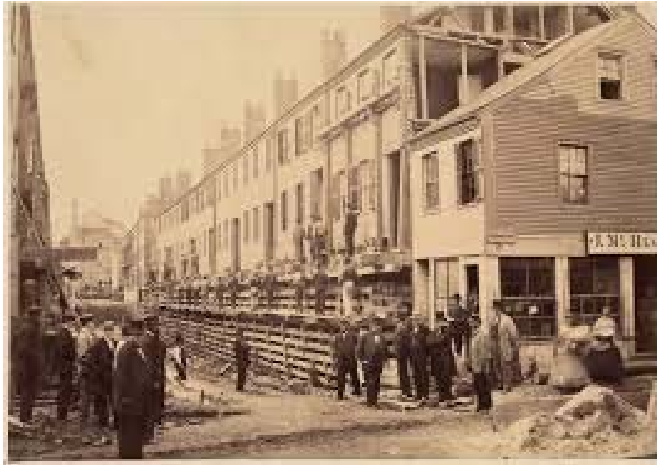
7. To relieve tidal flooding, the neighborhood's streets were raised in 1868
