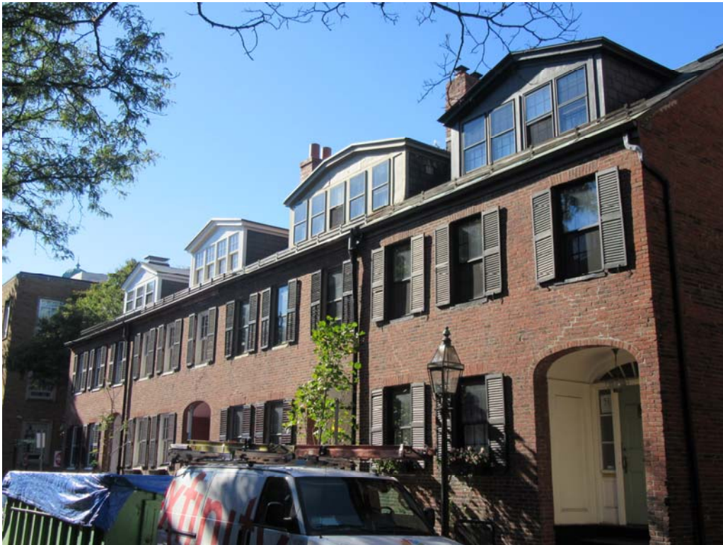
1. The Federal-style houses of Fayette Street are the oldest in Bay Village
