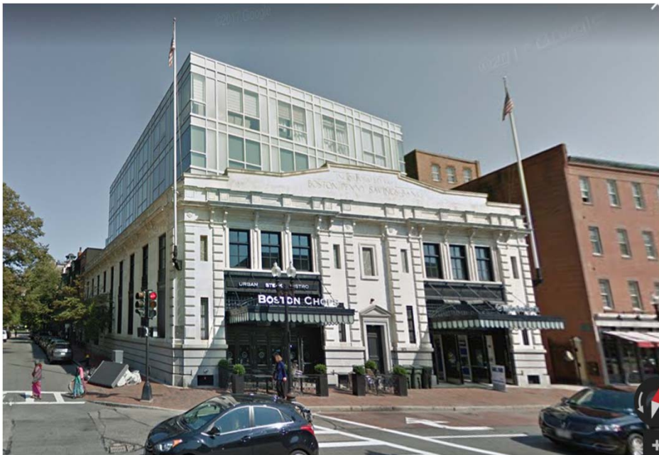
26. Though built on a South End rooftop, this setback addition appears to stand somewhere behind its historic neighbors
