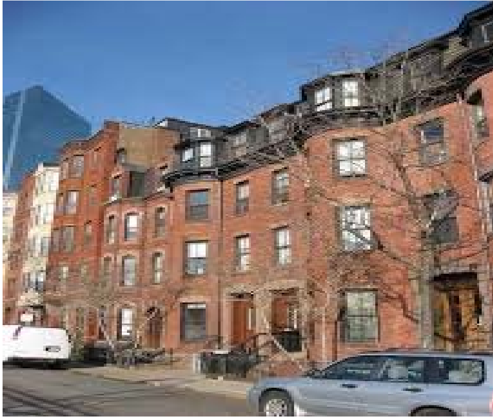
5. The bow-fronted rowhouses of Cortes Street resemble those of the South End
