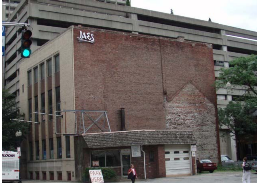
29. The much-altered former church and publishing house at 212 Stuart Street eventually became a restaurant
