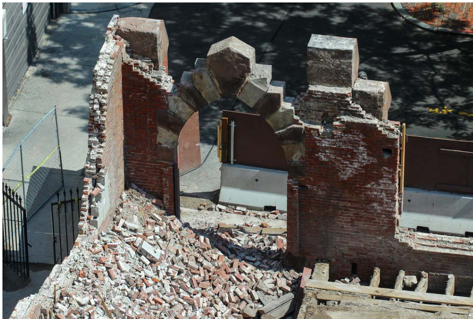
30. Demolition in progress
