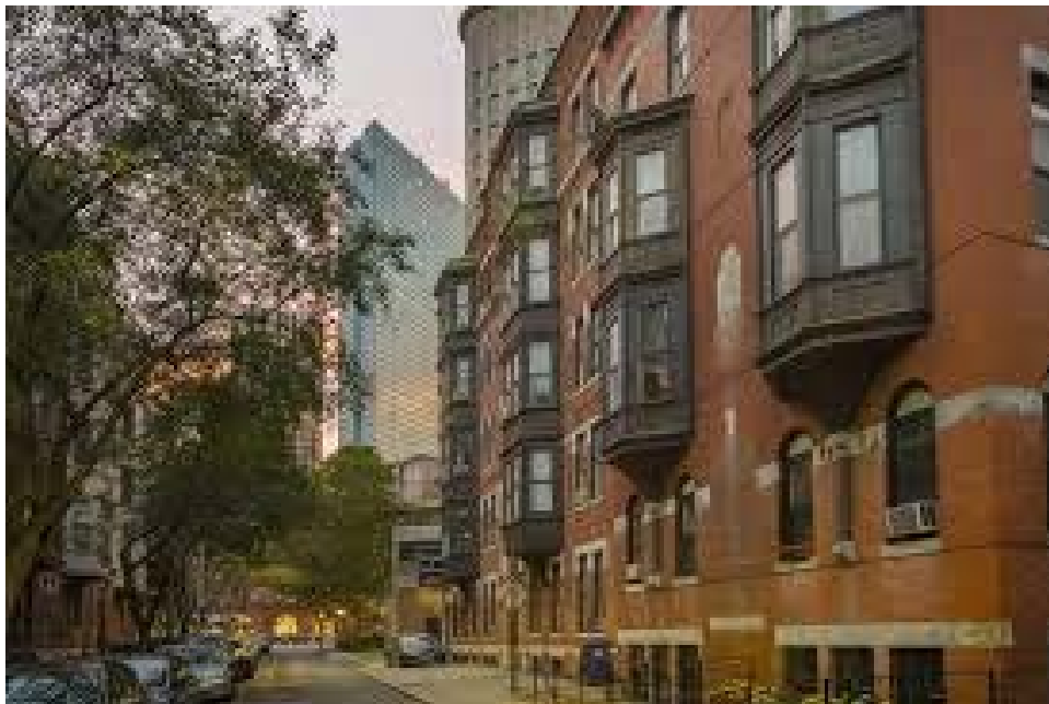
6. Ruskin Gothic-style apartment buildings on Isabella Street would be equally at home in the Back Bay
