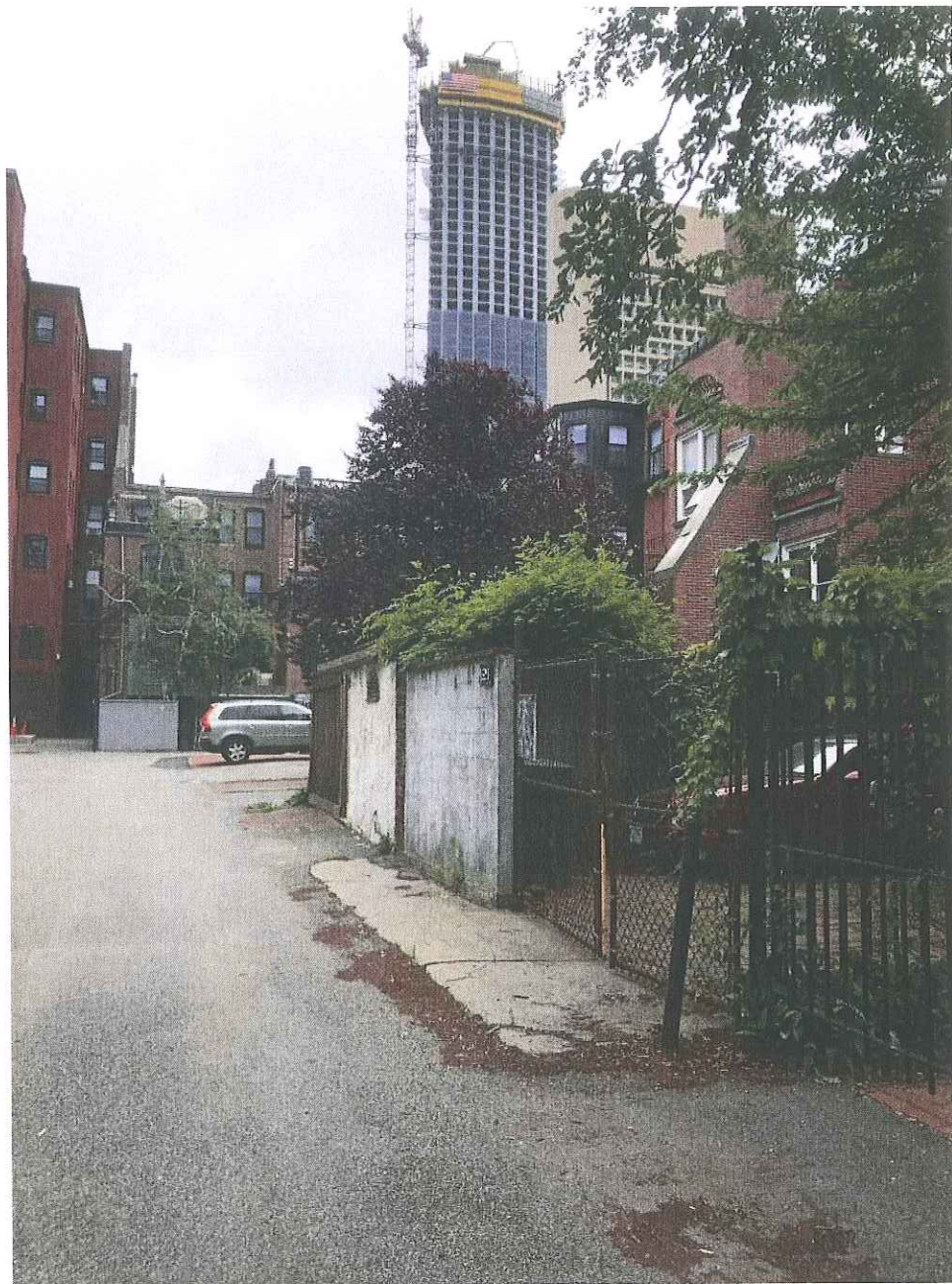
REAR ALLEY FACING NORTH
