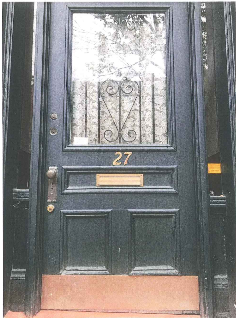
EXISTING FRONT DOOR
