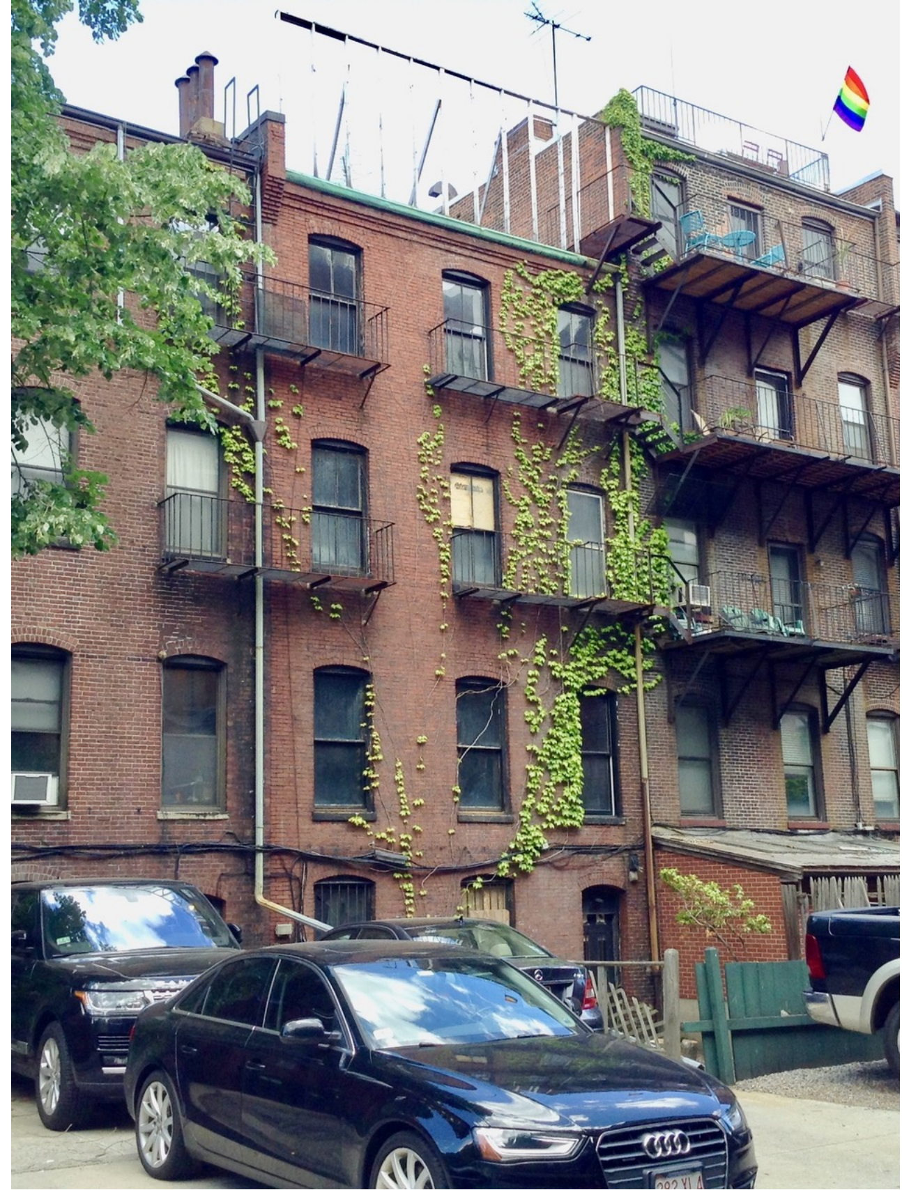
1 EXISTING SOUTH FACADE
