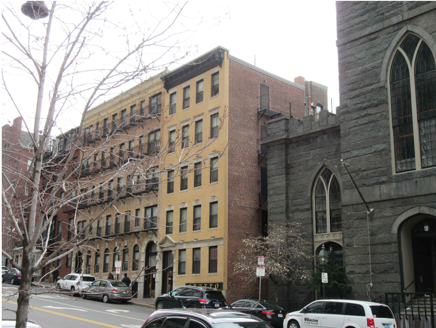
VIEW SOUTHWEST FROM BOWDOIN STREET (EQUIPMENT NOT VISIBLE)
