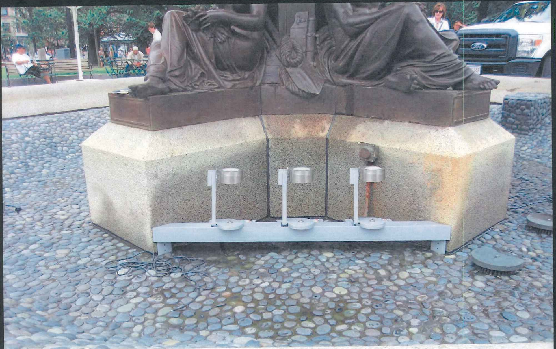
EARLIER DESIGN Note low water sensor conduit.
