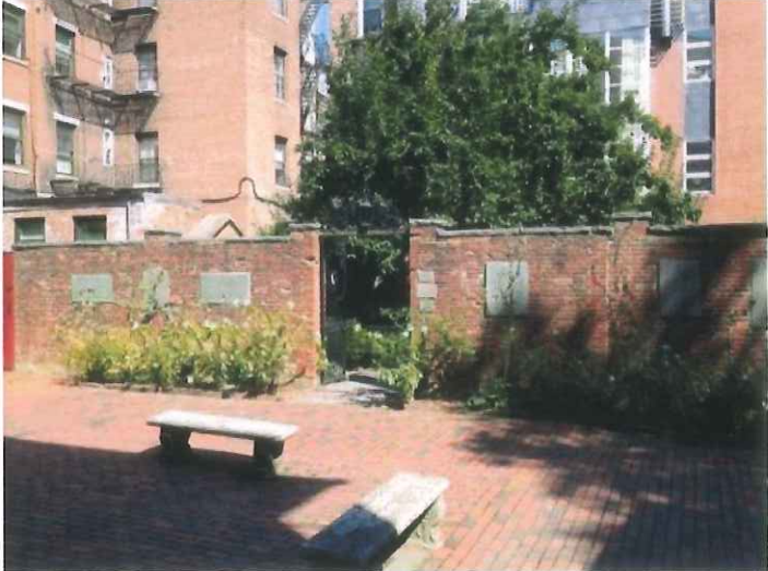
Existing Brick Walls with Historic Plaques
