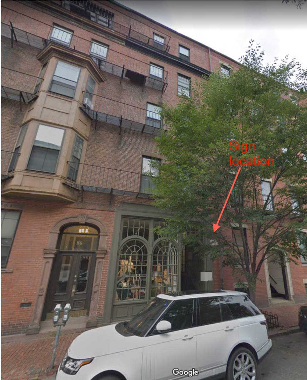
FULL BUILDING FACADE
