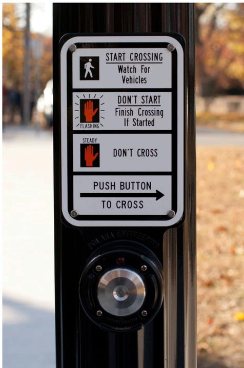
Vibrodetectable devices vibrate to communicate information through touch. Vibrodetectable arrows indicate when the **WALK** indication is in effect, and which direction to cross.
