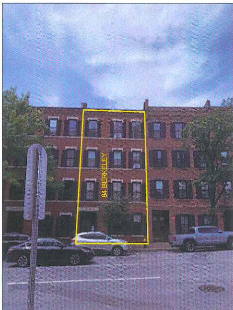
PHOTO C (DIRECTLY ACROSS BUILDING ON BERKELEY STREET)
