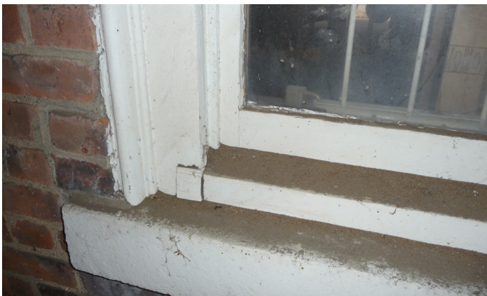
figure 11 | window B exterior sill Showing added window casing
