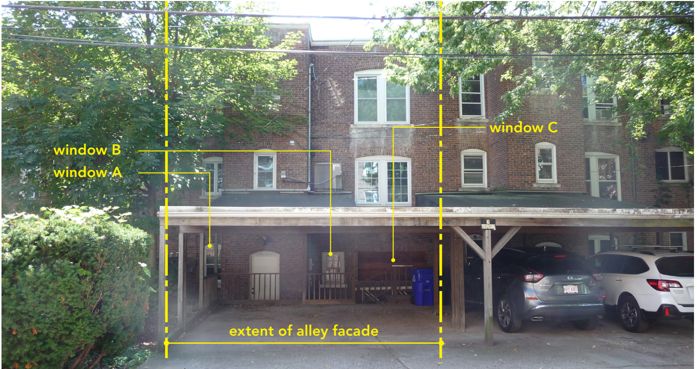
figure 3 | Private Alley Facade
