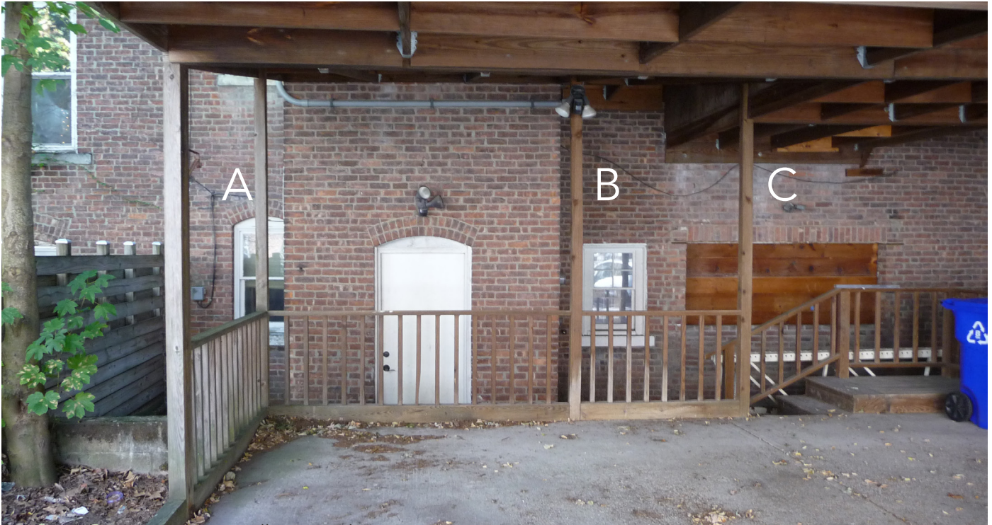
figure 15 | existing Private Alley Facade
