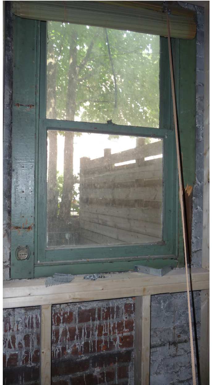
figure 6 | window A interior view
