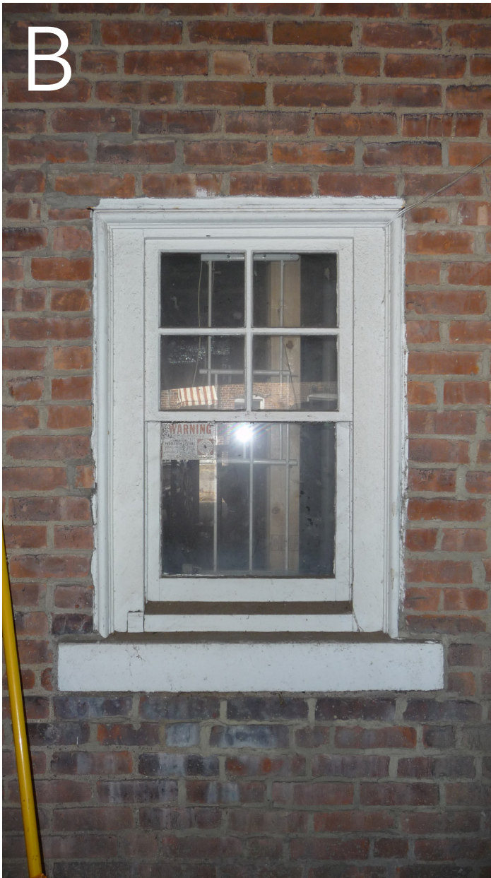
figure 9 | window B exterior view Showing added trim in addition to brick mold.
