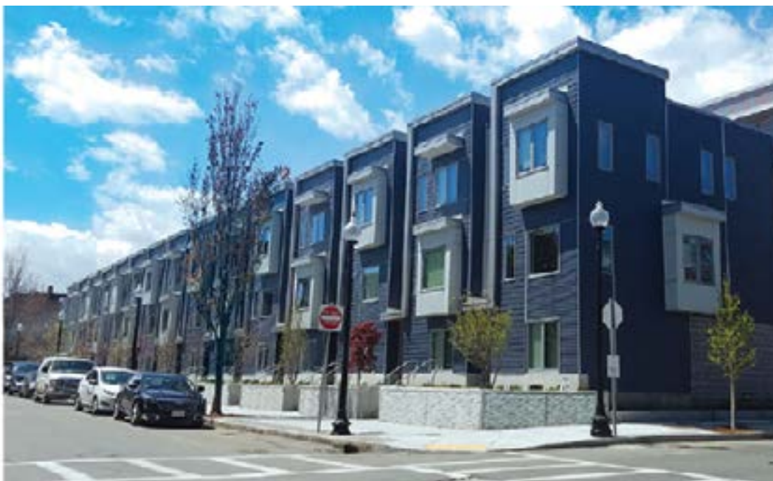
Coppersmith Village Homeownership, East Boston 8 income-restricted ownership units @ 80% AMI
