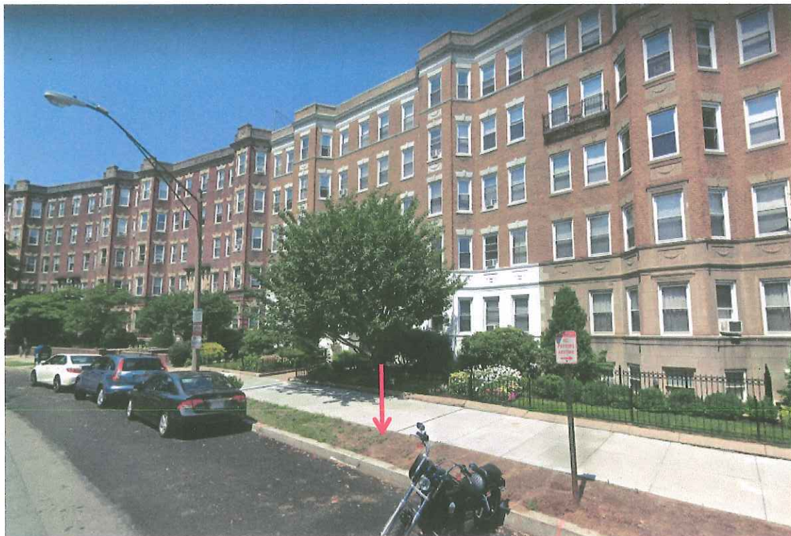
Proposed location of parking meter PD3 on Park Drive.
