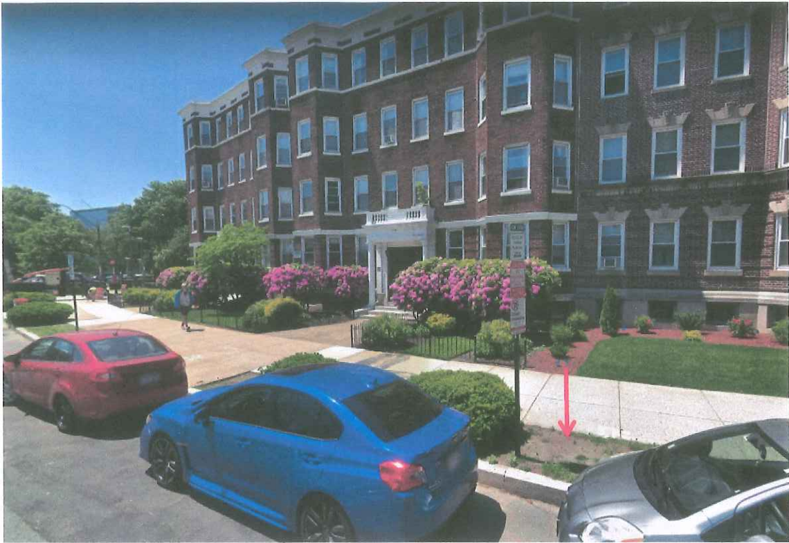
Proposed location of parking meter PD2 on Park Drive.
