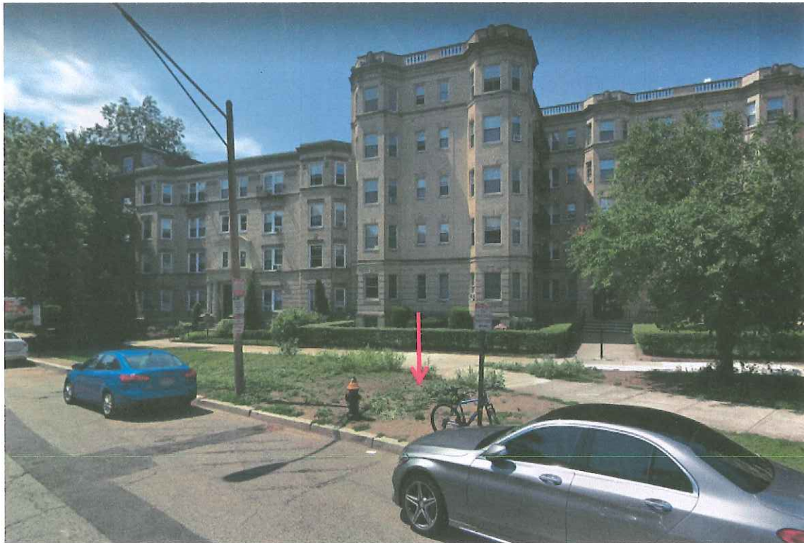
Proposed location of parking meter PD7 on Park Drive.
