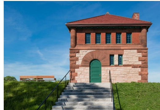
Fisher Hill Reservoir Gatehouse
