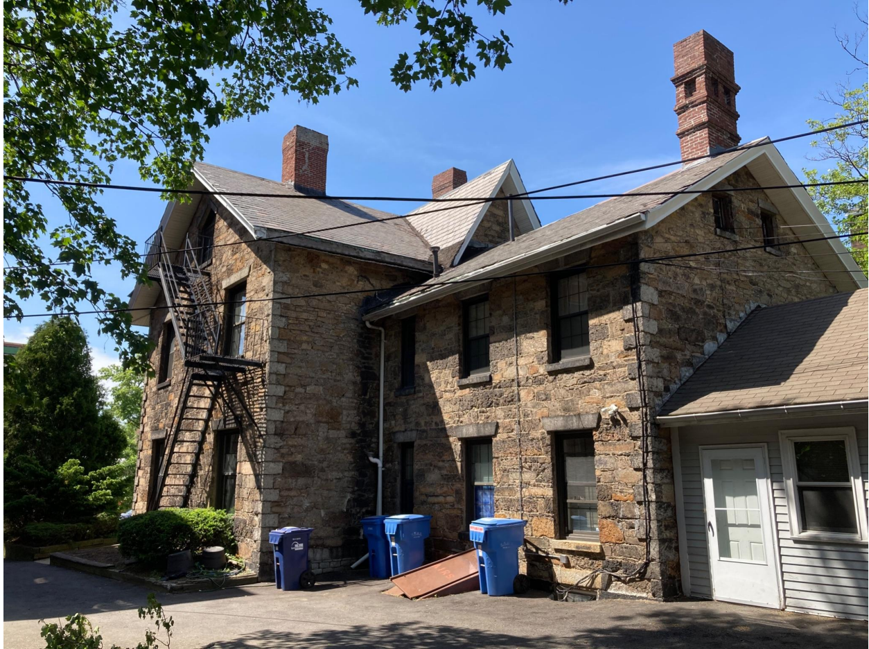
Figure 9: Rear of building (southeast corner)
