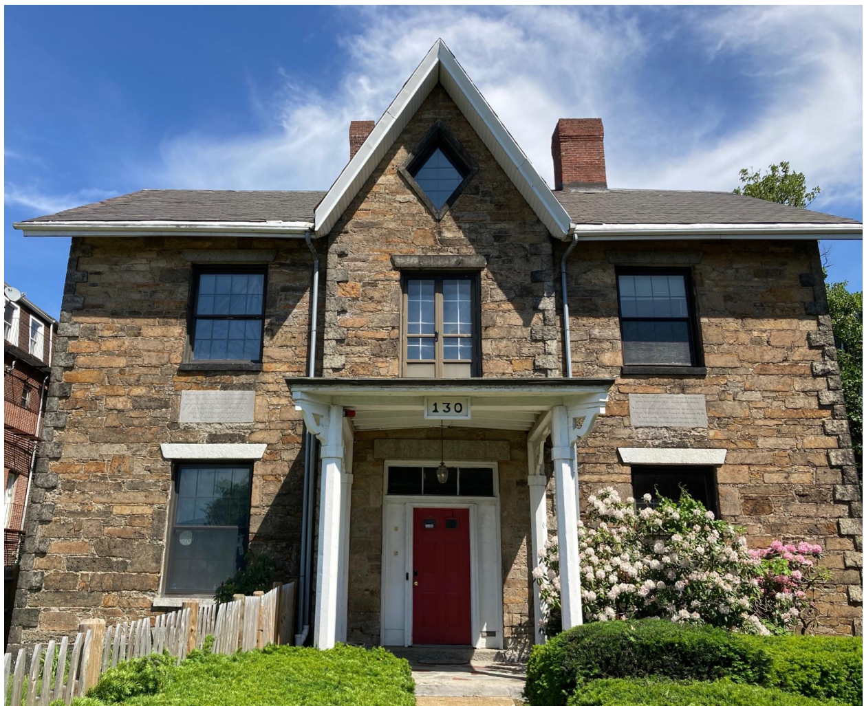
Figure 2: Entrance Front facade (west elevation)
