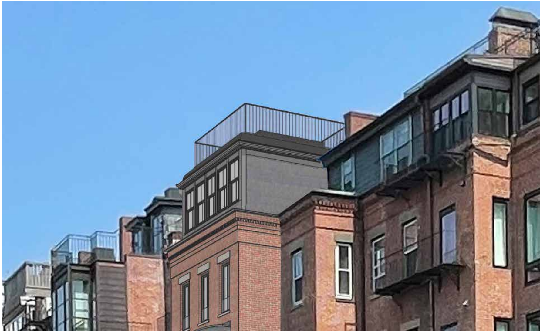
DETAIL VIEW FROM SHAWMUT AVENUE
