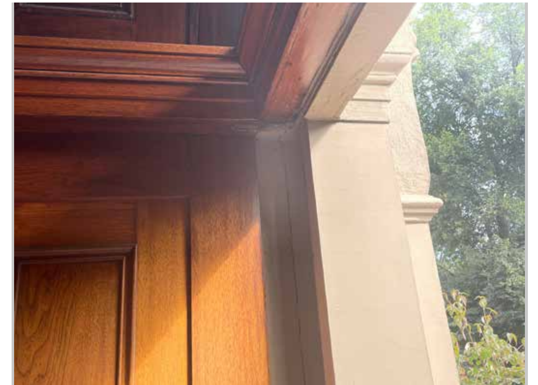
REMOVED WOOD DOOR JAMB
