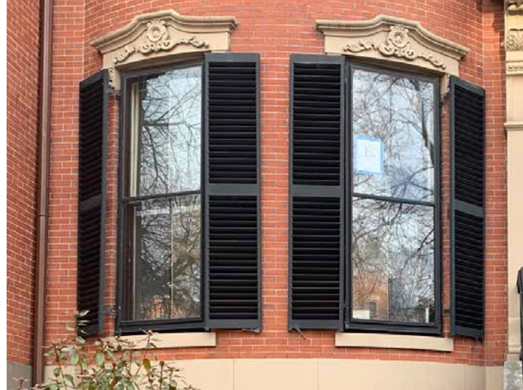
PARLOR LEVEL STORM WINDOWS
