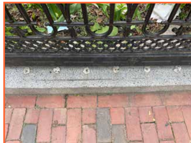
REPAIR HOLES IN GRANITE
