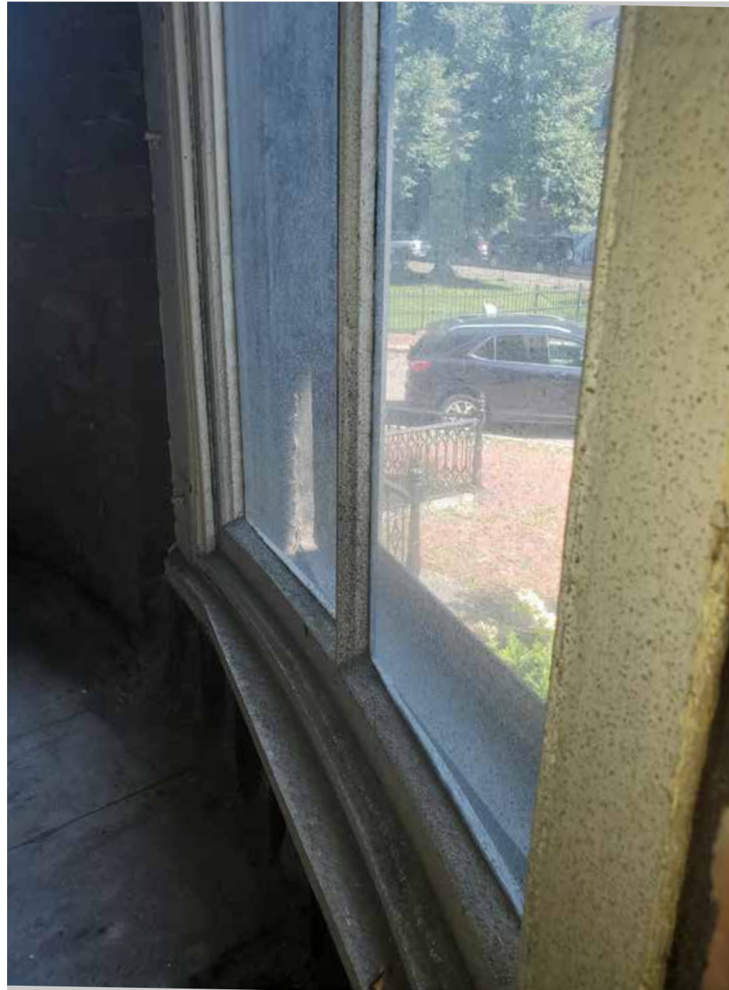
UNION PARK - PARLOR LEVEL WINDOWS
