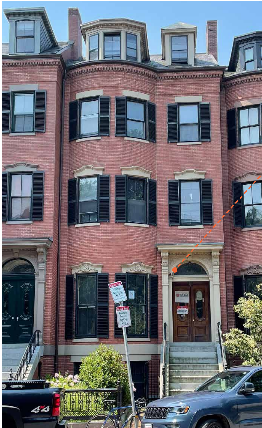
UNION PARK FAÇADE - EXISTING
