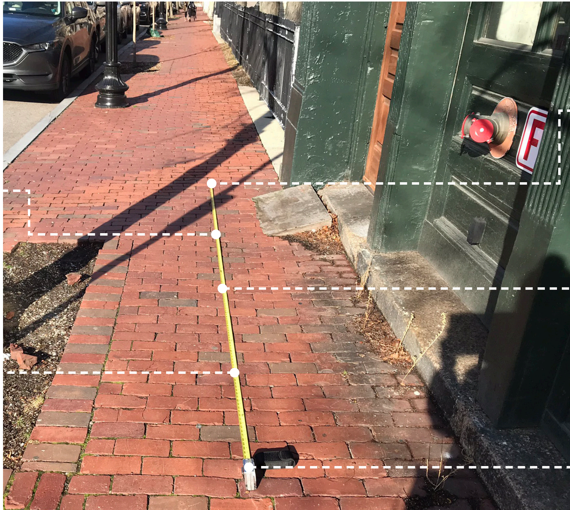
PITCH AWAY FROM BUILDING = 3.4° = 5.94% slope
