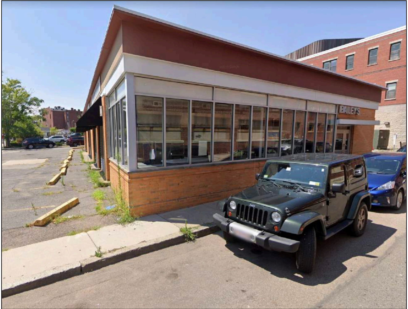
6. Existing side facade view along Palmer Street.
