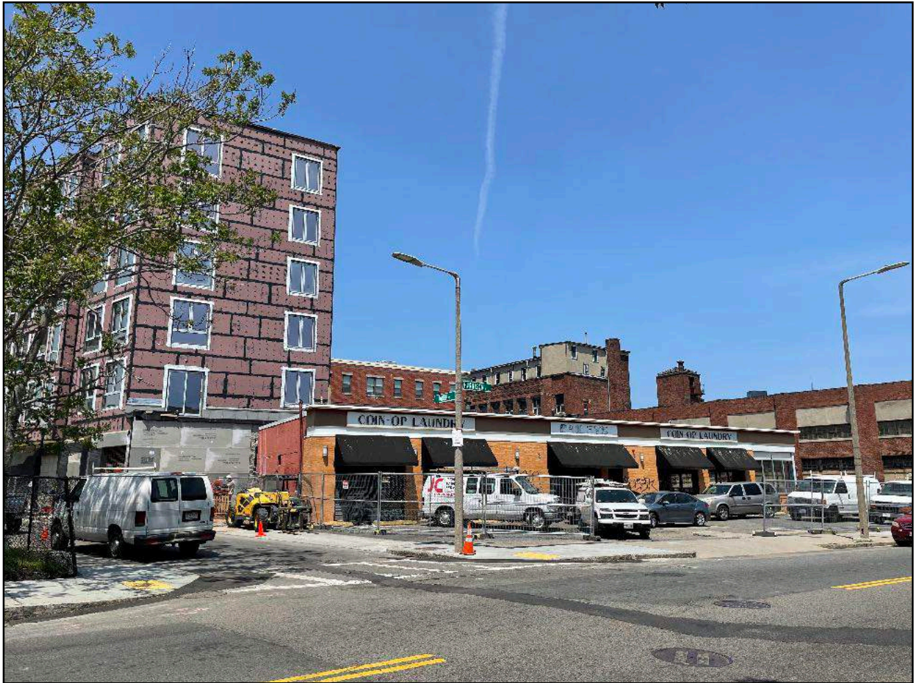
3. Existing view from Harrison Avenue and Taber Street with the #10 Taber adjacent new building.
