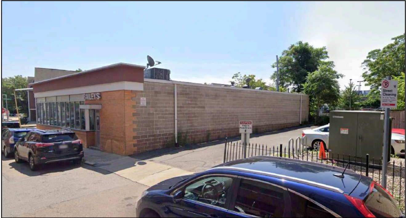
7. View of the existing rear side facade with cmu wall and existing driveway of adjacent building.
