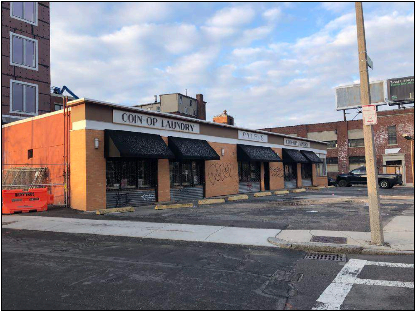
2. Existing building view from corner of Taber Street and Harrison Avenue.
