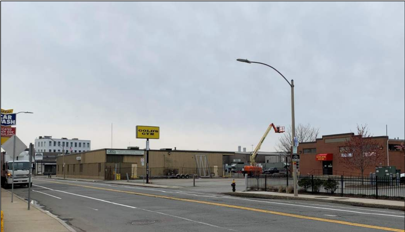
B6 – Northeast Elevation View From East Side of Dorchester Avenue
