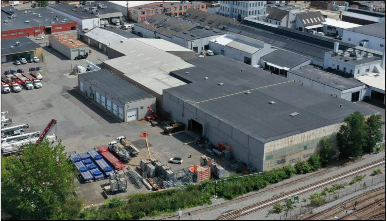
E7 – Northwest Elevation Aerial View from Above Western Abutting Train Tracks
