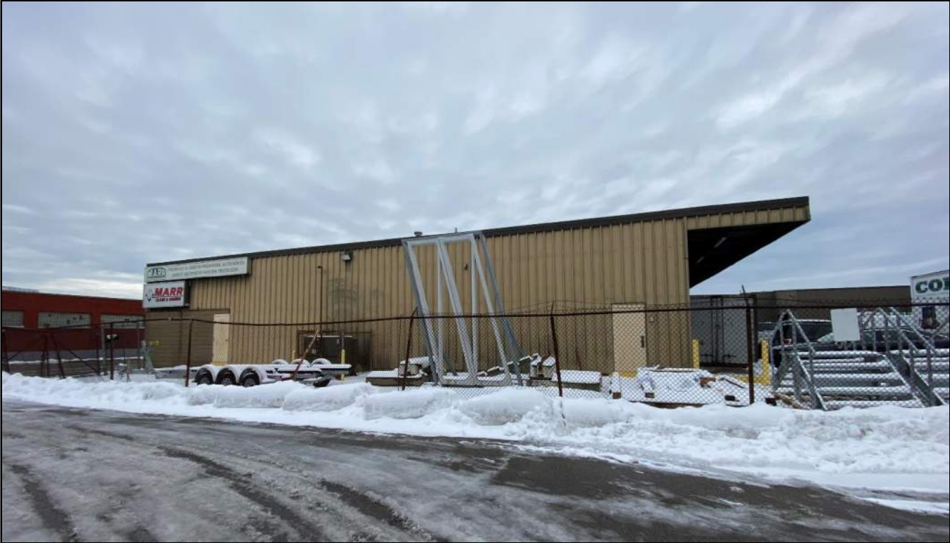
B1 – North Elevation View From Gold’s Gym Parking Lot
