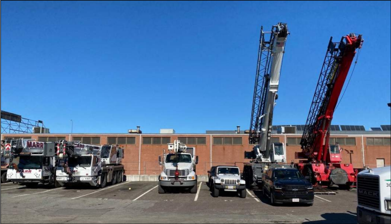
A5 – South Elevation View From Marr Crane & Rigging Parking Lot
