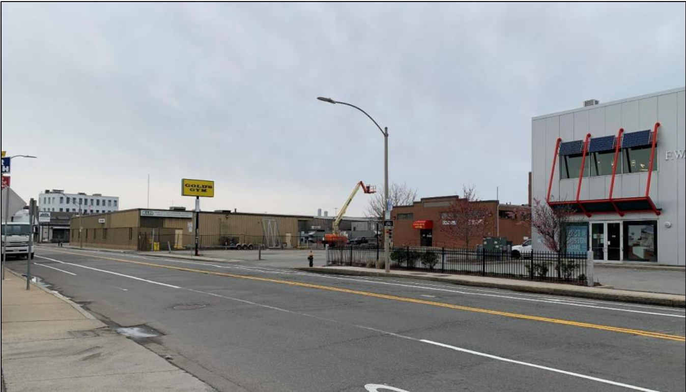
A6 – Northeast Elevation View From East Side of Dorchester Ave
