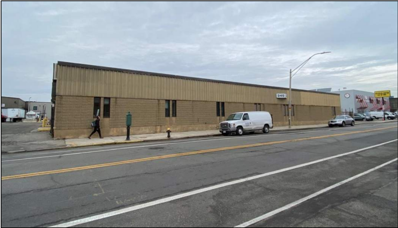
B4 – East Elevation View From East Side of Dorchester Avenue
