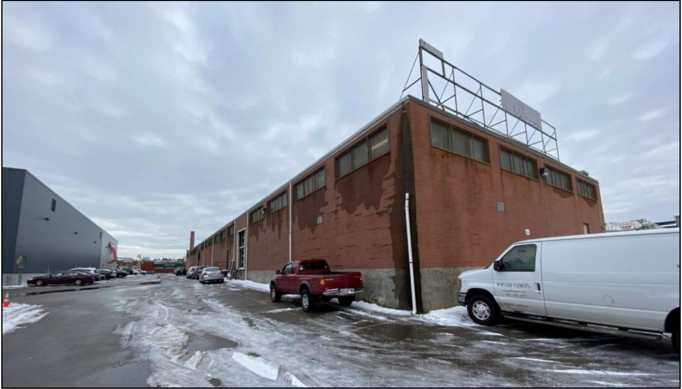
A3 – Northwest Elevation View From Rear Driveway/Train Tracks
