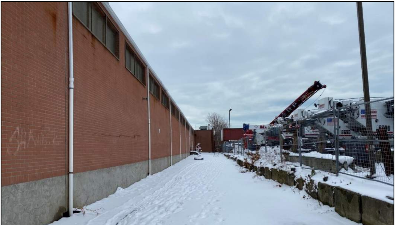
A4 – South Elevation Southern Façade Looking East
