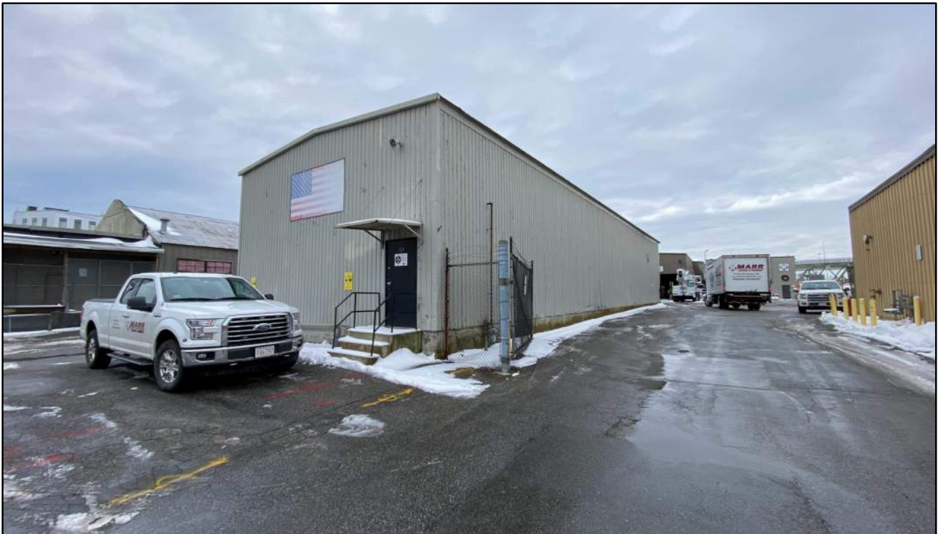
D2 – Northeast Elevation View from Northeast Access Drive from Dorchester Avenue
