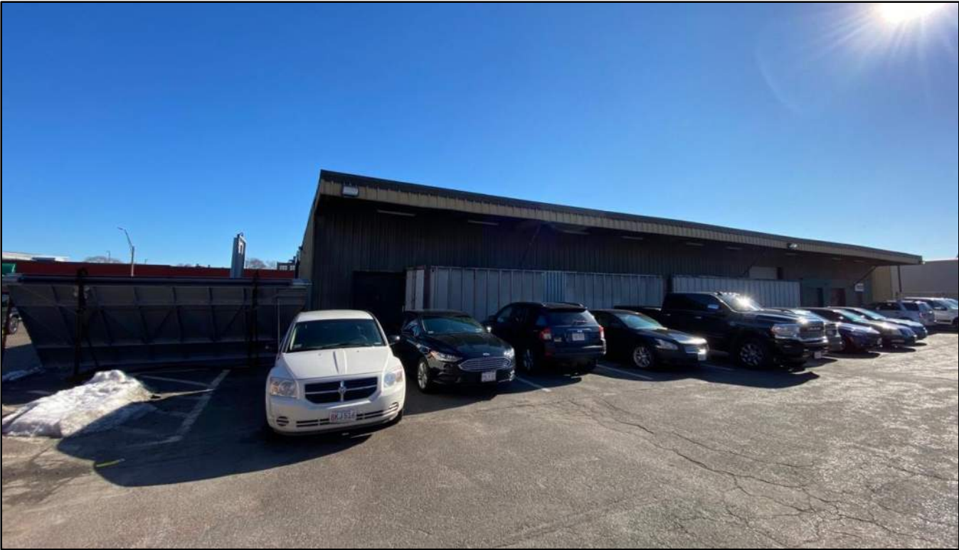
B2 – West Elevation View From Marr Crane & Rigging Parking Lot
