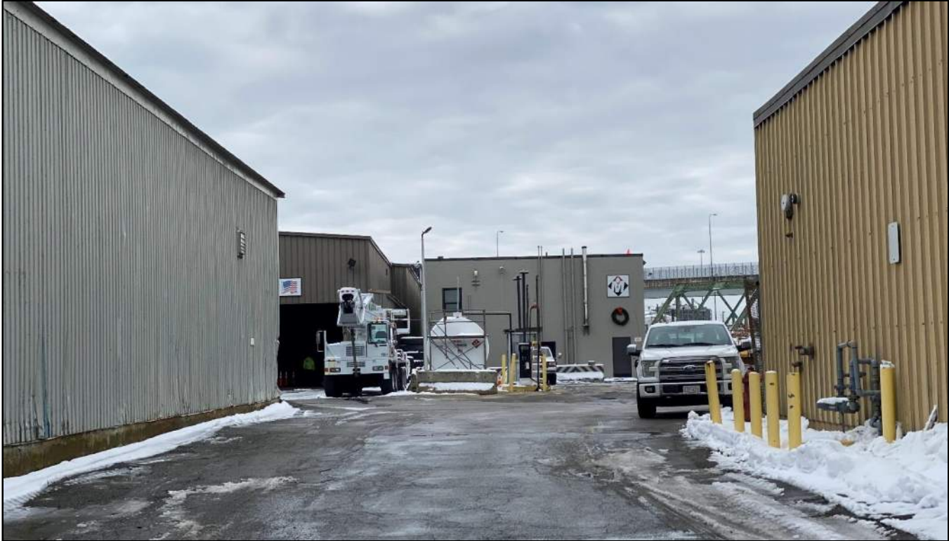
C1 – East Elevation View from Dorchester Ave, Between Metal Shed & 345 Dorchester Ave
