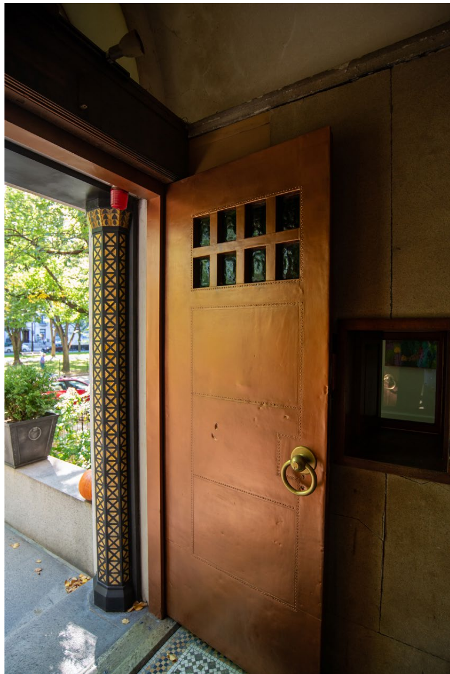
Copper clad entry doors
