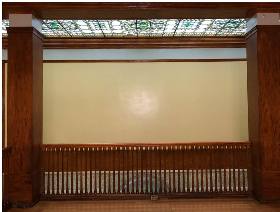
Looking east at apse overlook and skylight
