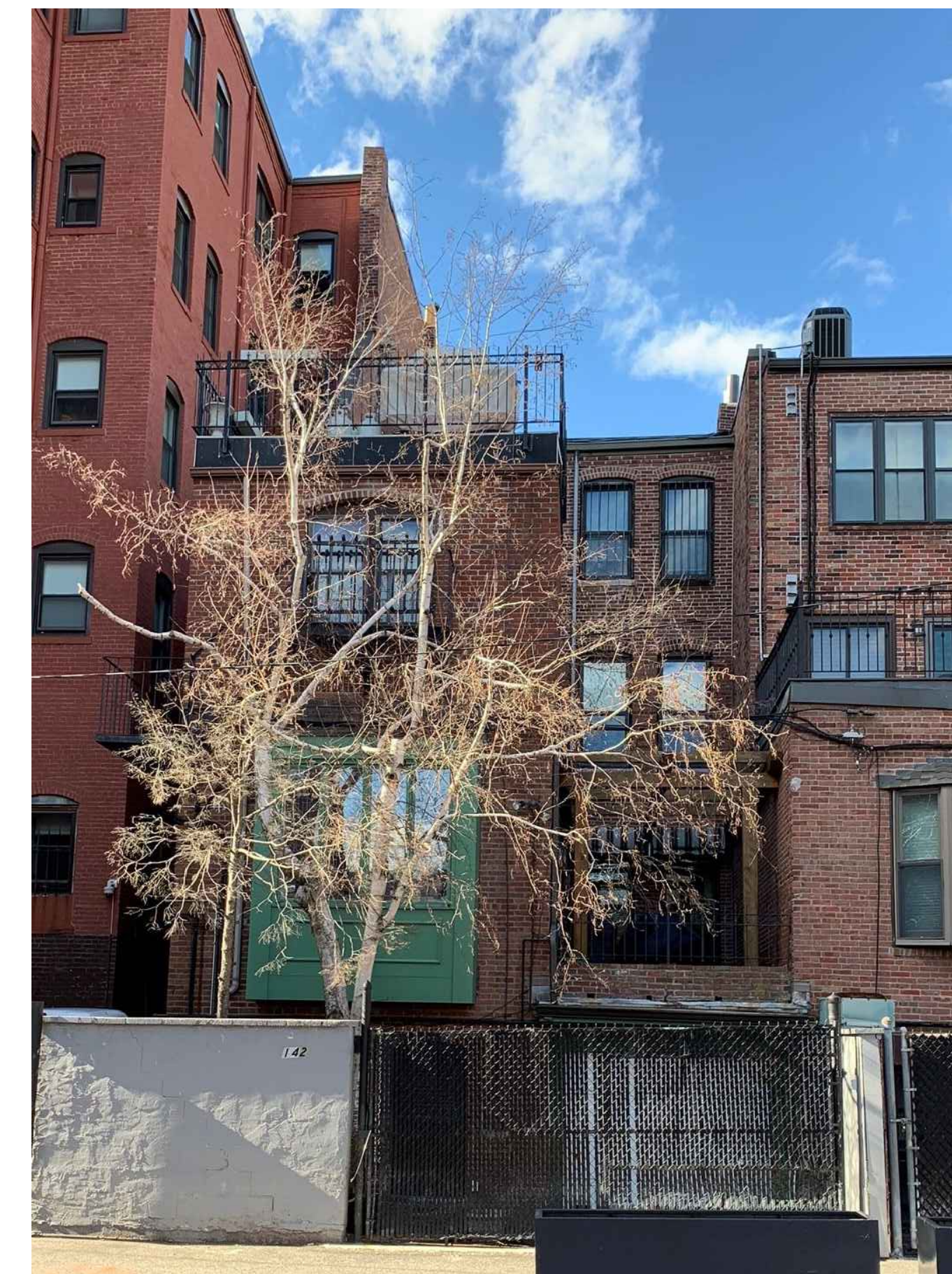
4 EX2.1 ST BOTOLPH ST. (SE) ELEVATION PHOTOGRAPH SCALE: NOT TO SCALE
