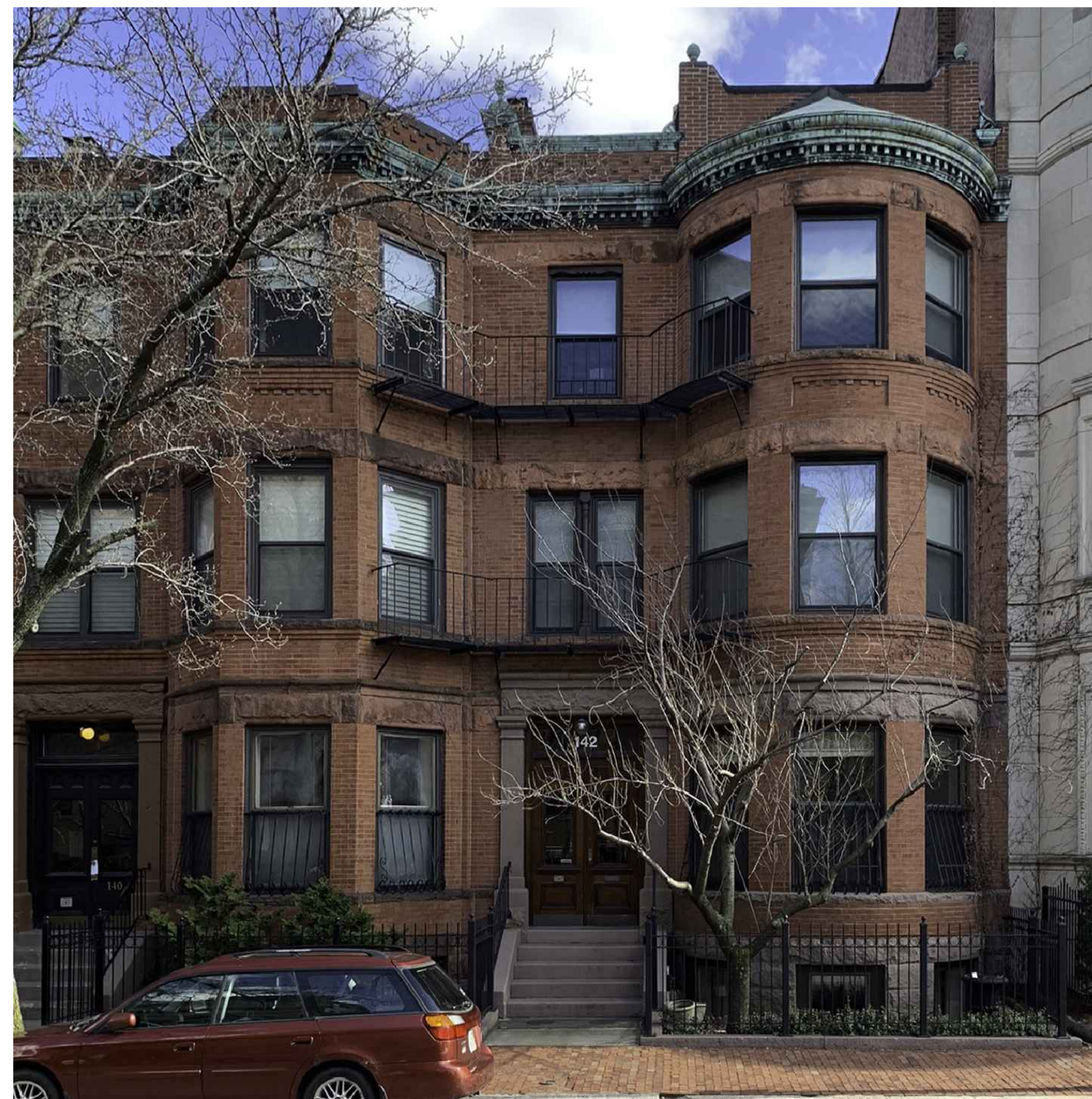
2 EX2.1 ST BOTOLPH ST. (NW) ELEVATION PHOTOGRAPH SCALE: NOT TO SCALE
