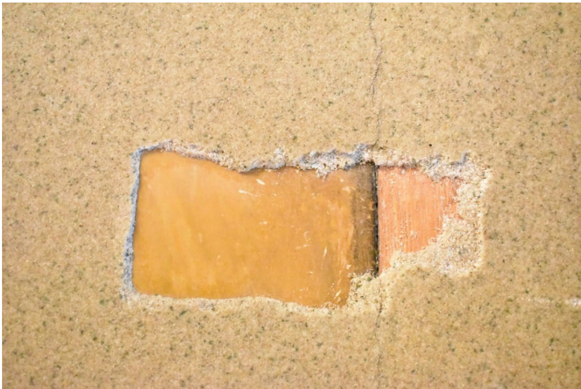
Photo 11. Inner Vestibule, wall detail showing original marble under covering, view east.
