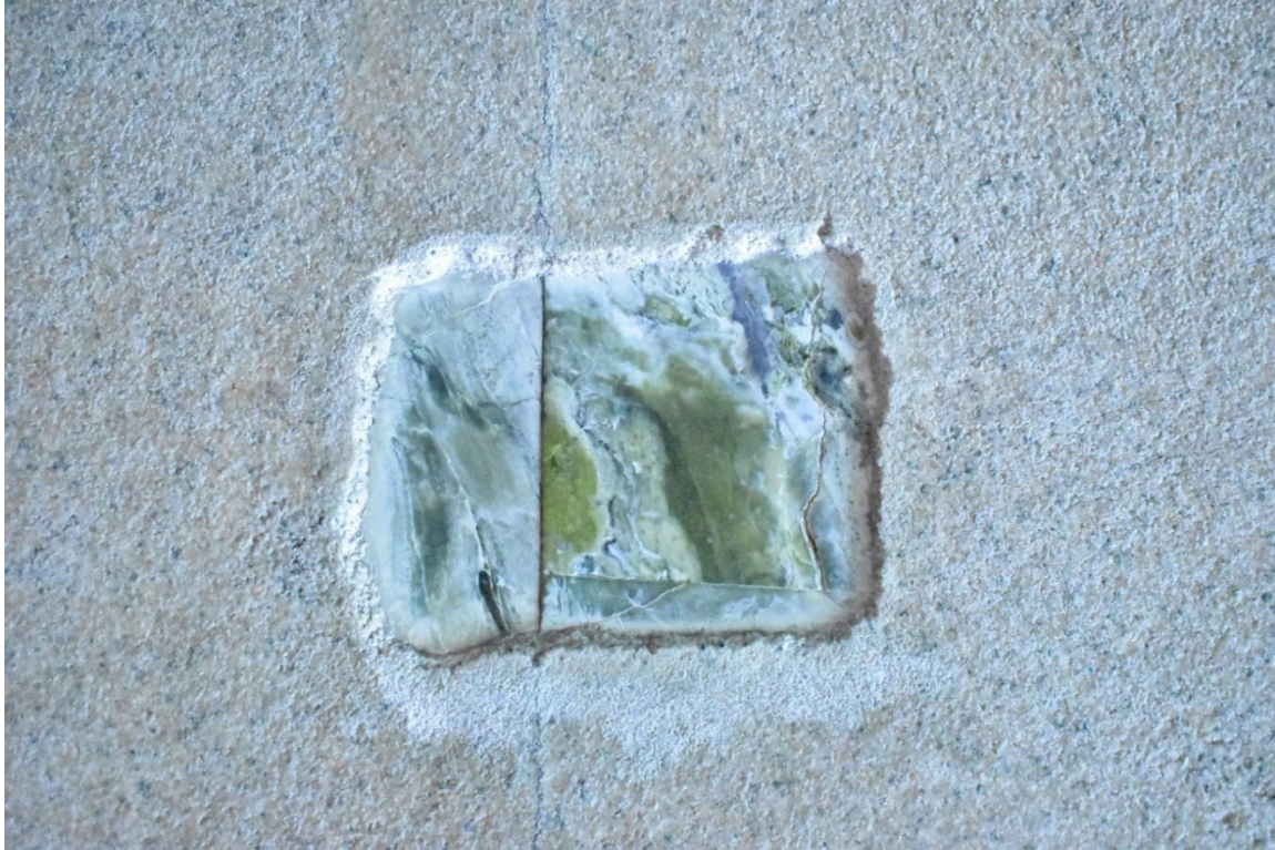
Photo 10. Outer Vestibule, wall detail showing original marble under covering, view east.
