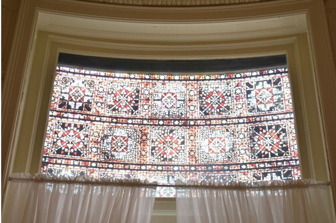
Photo 32. Drawing Room, stained-glass window plastic sheet reproduction detail, view south.
